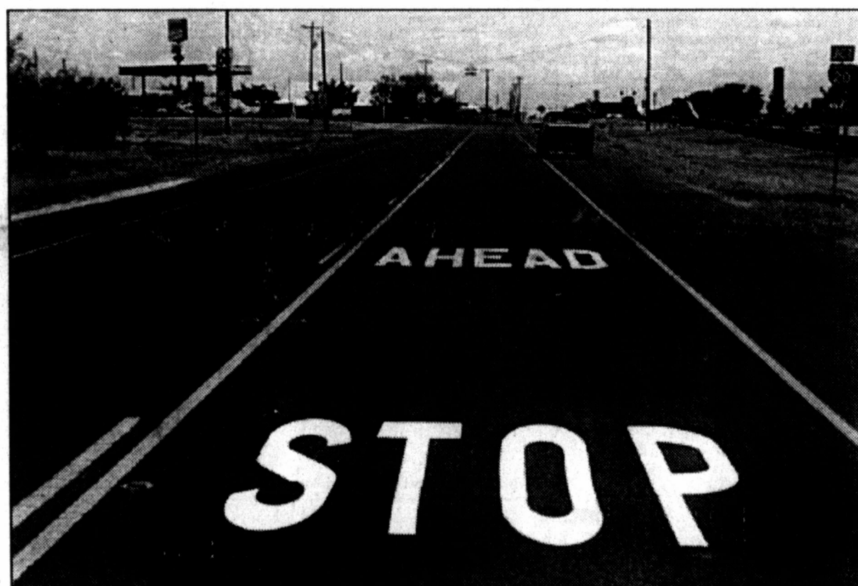
A SAFER SOUTH HWY. 208 is the goal of a new caution approaching the 208-East Hwy. 80 intersection in southeastern C-City. Rumble strips, "Cross Traffic Does Not Stop" signs and bigger yellow and red flashing lights will be added in coming weeks.
