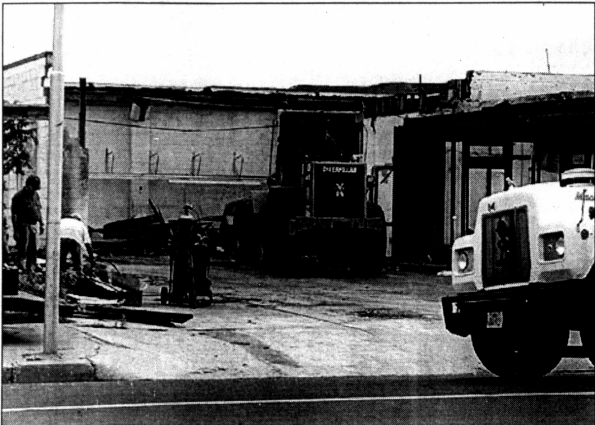
DEMOLITION MEN from the city were tearing down the old Britton's Diesel building at Oak and West Second Street Friday, cutting rebar with cutting torches and removing the debris in city trucks to the landfill.
