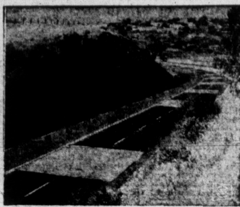
NEW ROAD ALERTS DRIVERS —Paving surfaces which "talk back" to the driver are helping to cut accidents along old U.S. 40 in California. The areas are called "rumble strips," and are squares of small stones glued to the road. They alert drivers to changing road conditions with an increased sound and a different "feel" of the road beneath the wheels. Where used, accidents have decreased by half.
