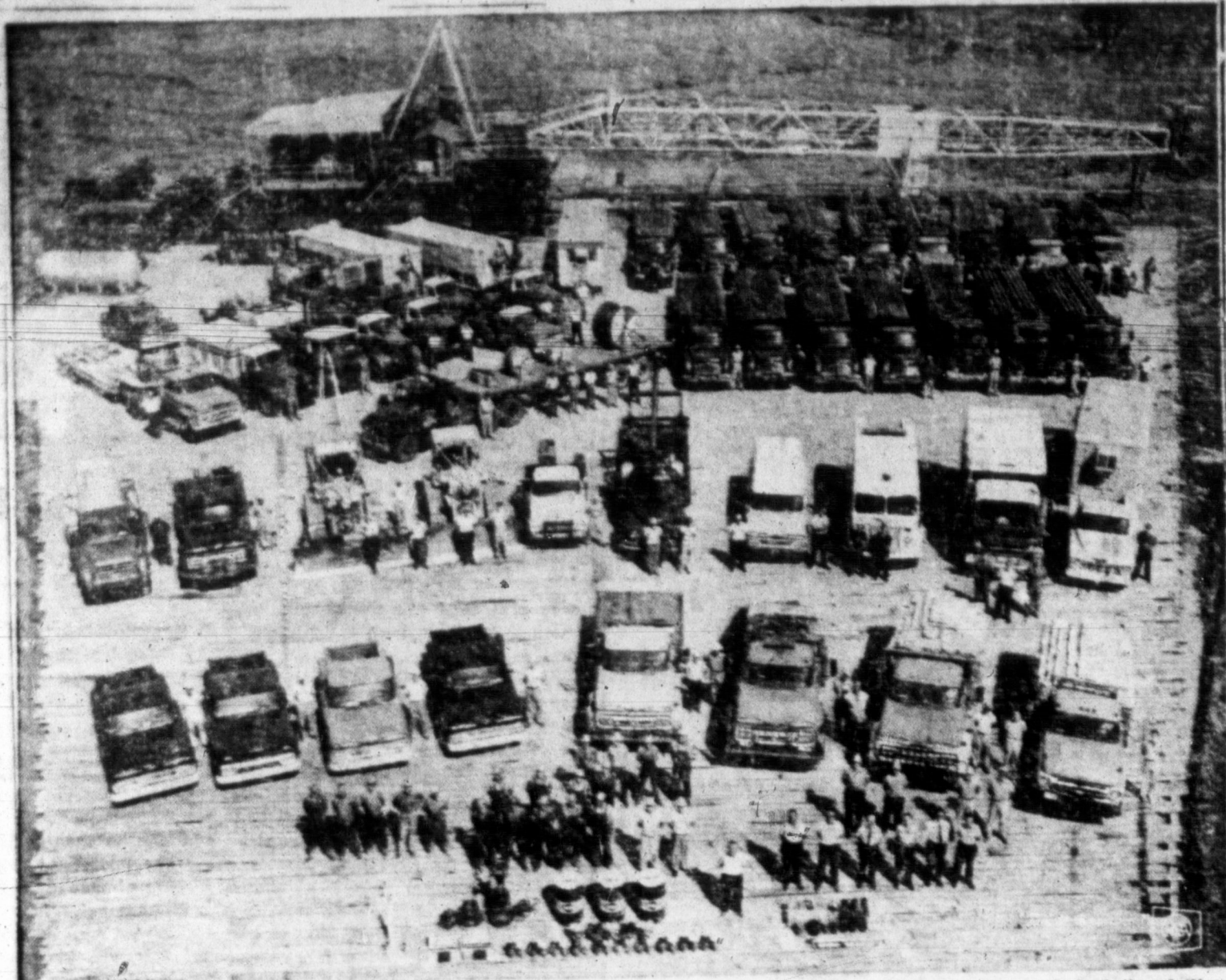
OIL WELL, ANYONE? —So you've always wanted to strike oil in the back yard? Gathered above, in one of the most unusual field photographs ever taken, is just about everything you'd need to bring a typical oil well into being. Assembled in southern Mississippi is McCormick Field Unit 26-1 of the Sun Oil Co.—88 men and almost $1.5 million in
