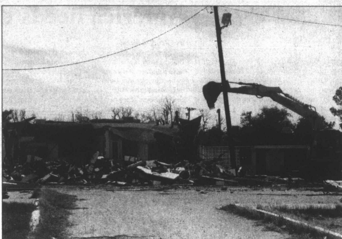
MAKING WAY FOR THE FUTURE – Crews from Ellis Construction were hard at work Tuesday beginning demolition of the old Mitchell County Hospital buildings, located on Chestnut Street. The deteriorating condition of the structure required demolition as a matter of safety.
