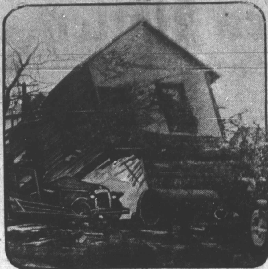
This photo shows a garage-apartment in Miami, Fla., which was raised clear of its foundation by the force of the recent hurricane and left resting on a touring car that had been parked beside it.
