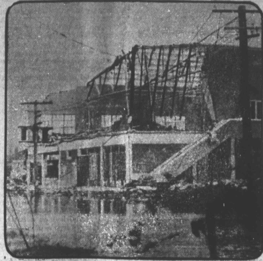
This shows a theater building in Miami, Fla., literally ripped apart by the recent hurricane. The top and front were torn off and carried into the next block, leaving only a shell. Note how the street in front is flooded.
