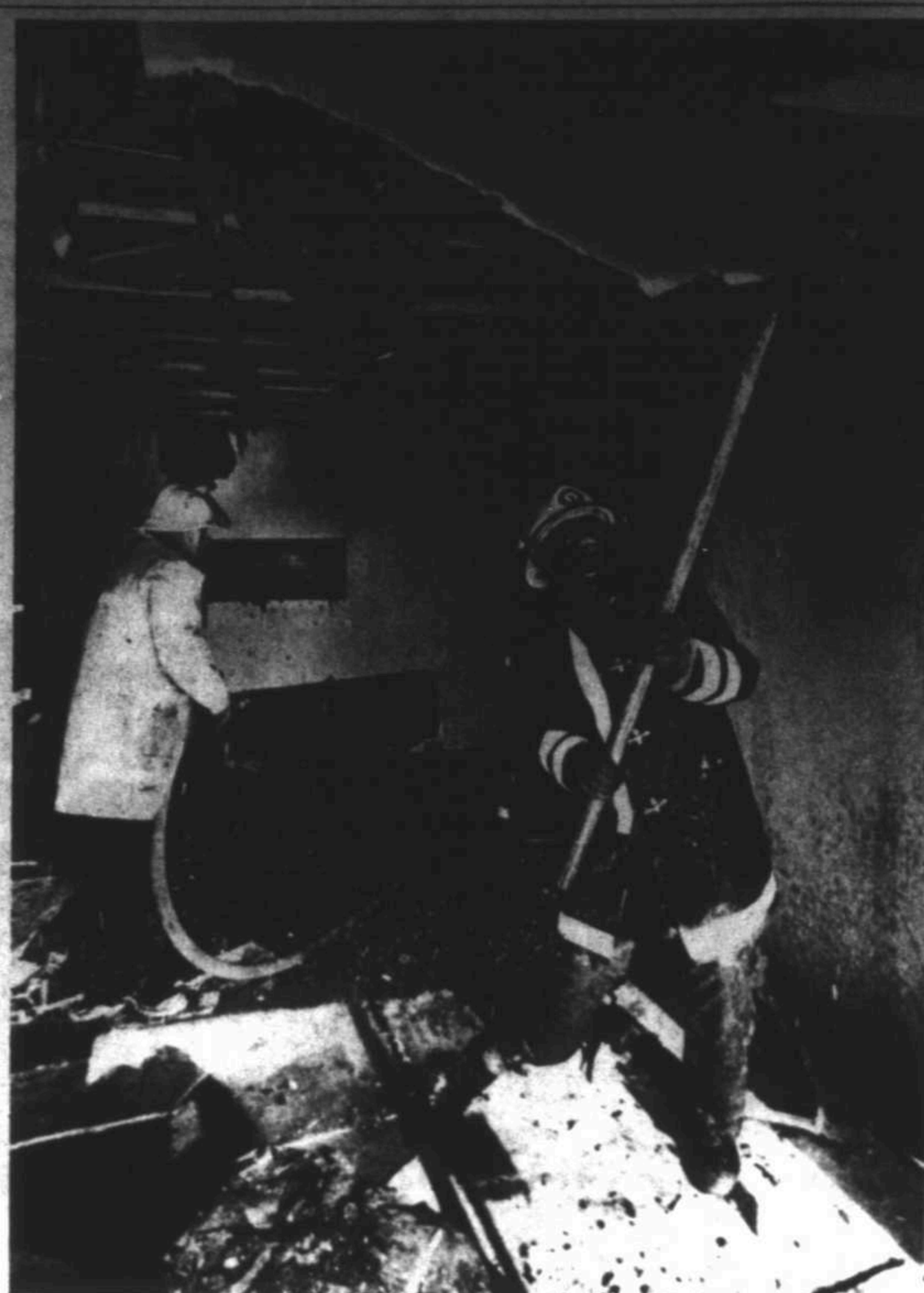
Firemen work to put out a blaze that heavily damaged 12 units of the Oakridge apartment complex under construction at 4400 Holiday Hill Road. Cause of the fire, which broke out about 11 a.m. Monday and took 49,000 gallons of water to extinguish, is under investigation by the Midland fire marshal's office. A spokesman said arson is suspected.
