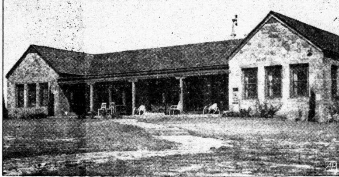
Red sand stone from Ector County's old courthouse, auctioned for $1, was used in the construction of this palatial ranch home in Northwest Crane county. It is owned by Glen Allen and is valued, with furnishings, at $50,000. It also serves as headquarters for the 35,000-acre Allen ranch, which covers the corners of Crane, Ward, Ector and Winkler counties.
