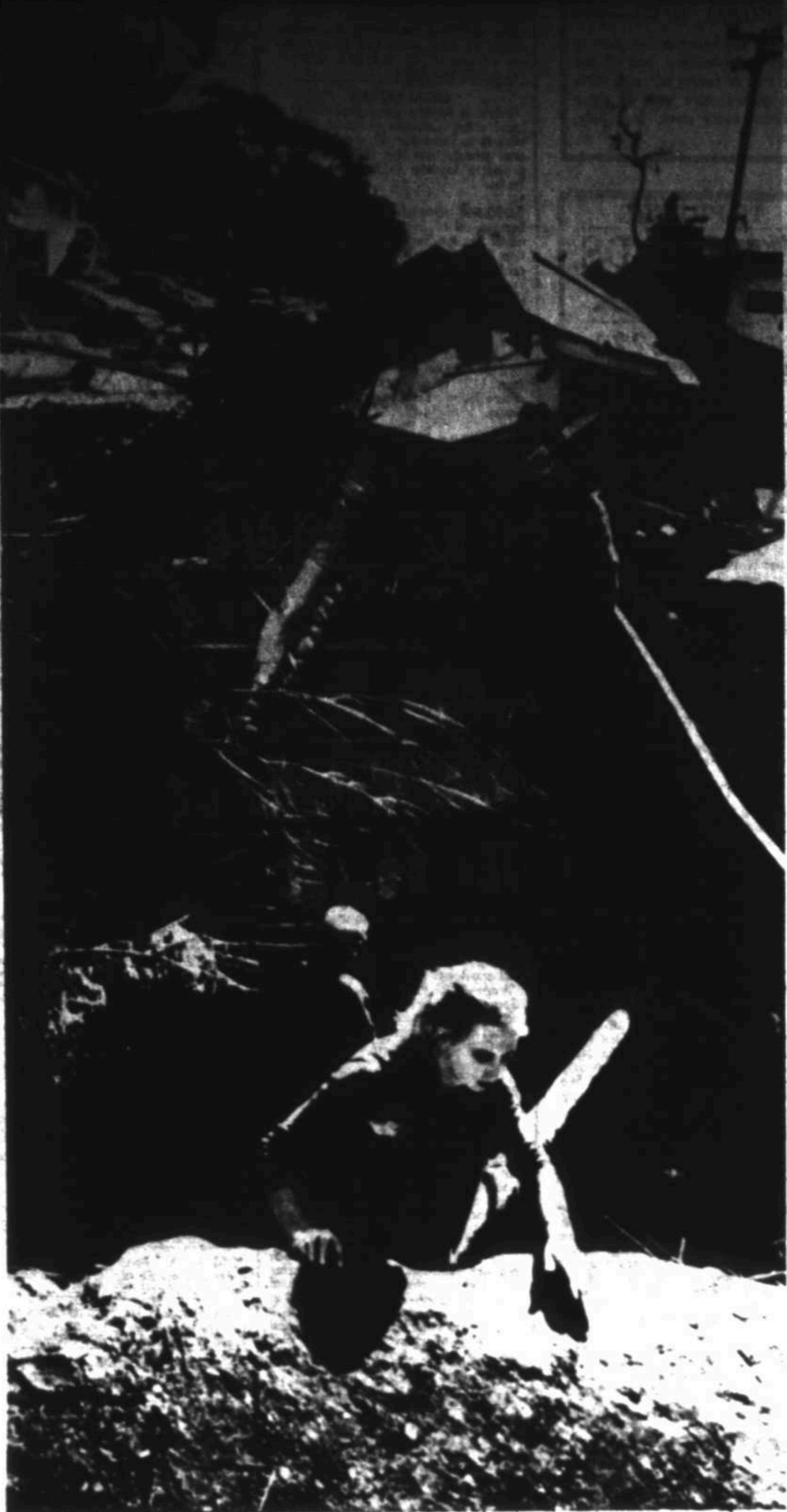
Aptos, Calif., resident Alix Wall, 28, climbs out of what was Spreckles Road. A man in the backgrounds follows Miss Wall's route: climbing down the collapsed deck of a house into the hole, balancing on a fallen telephone pole to "cross the street," then crawling up onto the shoulder.
