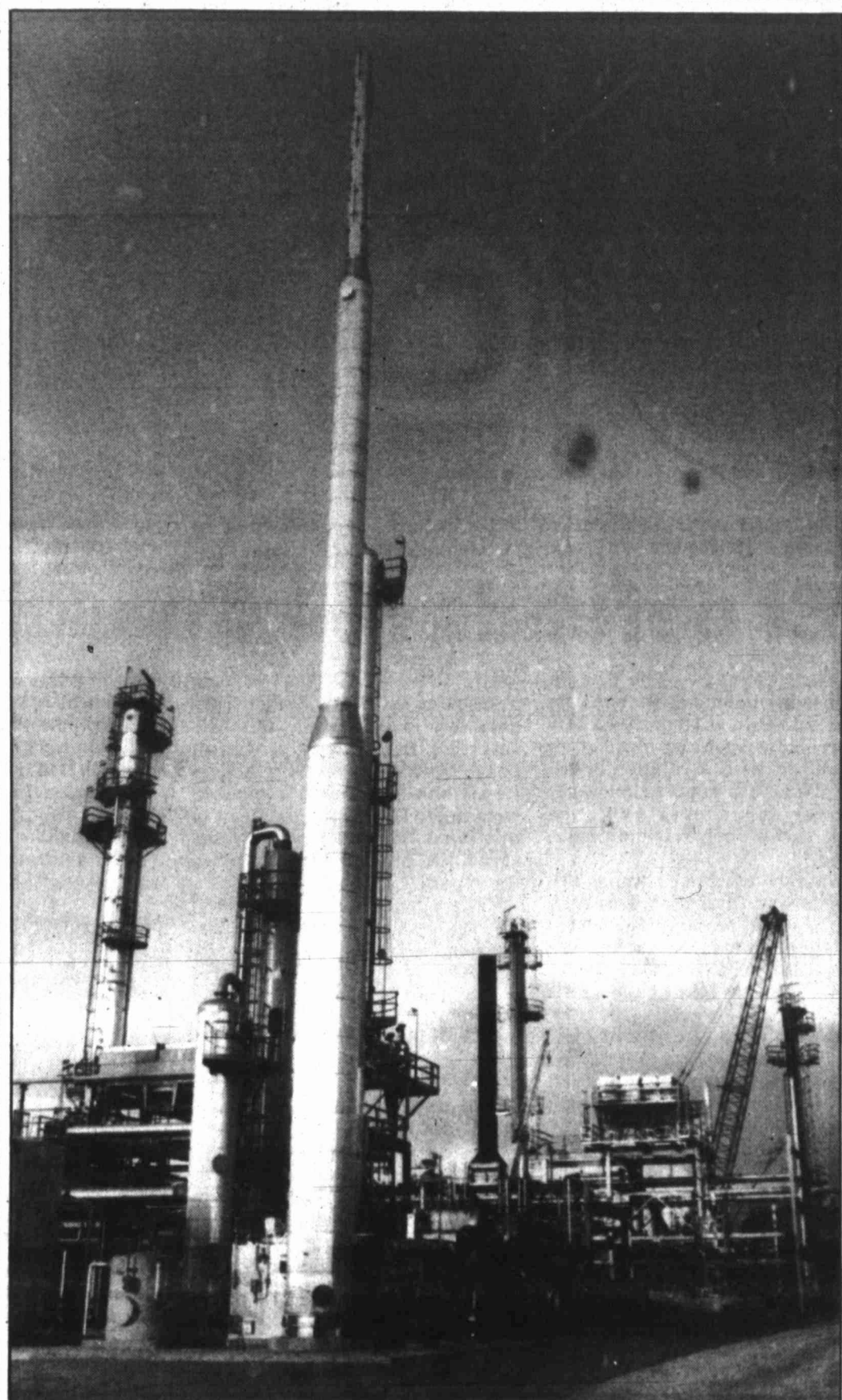
New towers rise into the air as part of the low sulfur diesel unit at the Fina Refinery. The reactor vessel for the unit will be set into place Thursday, with the unit scheduled to be placed online in July.
