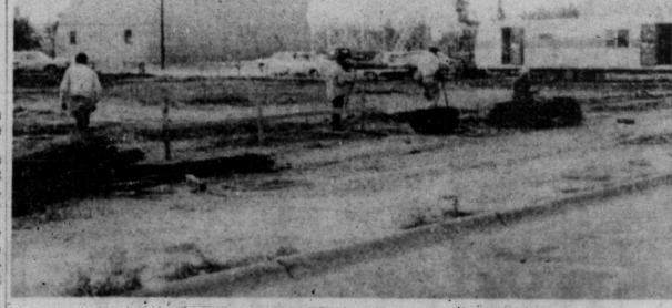
POST OFFICE CONSTRUCTION BEGINS —Excavation has been completed on the new Post Office construction project here as workmen prepare for the foundation of the building. The new structure will be located at Avenue R and Twenty-fourth Street, about 1 1/2 blocks south of the present Post Office.
