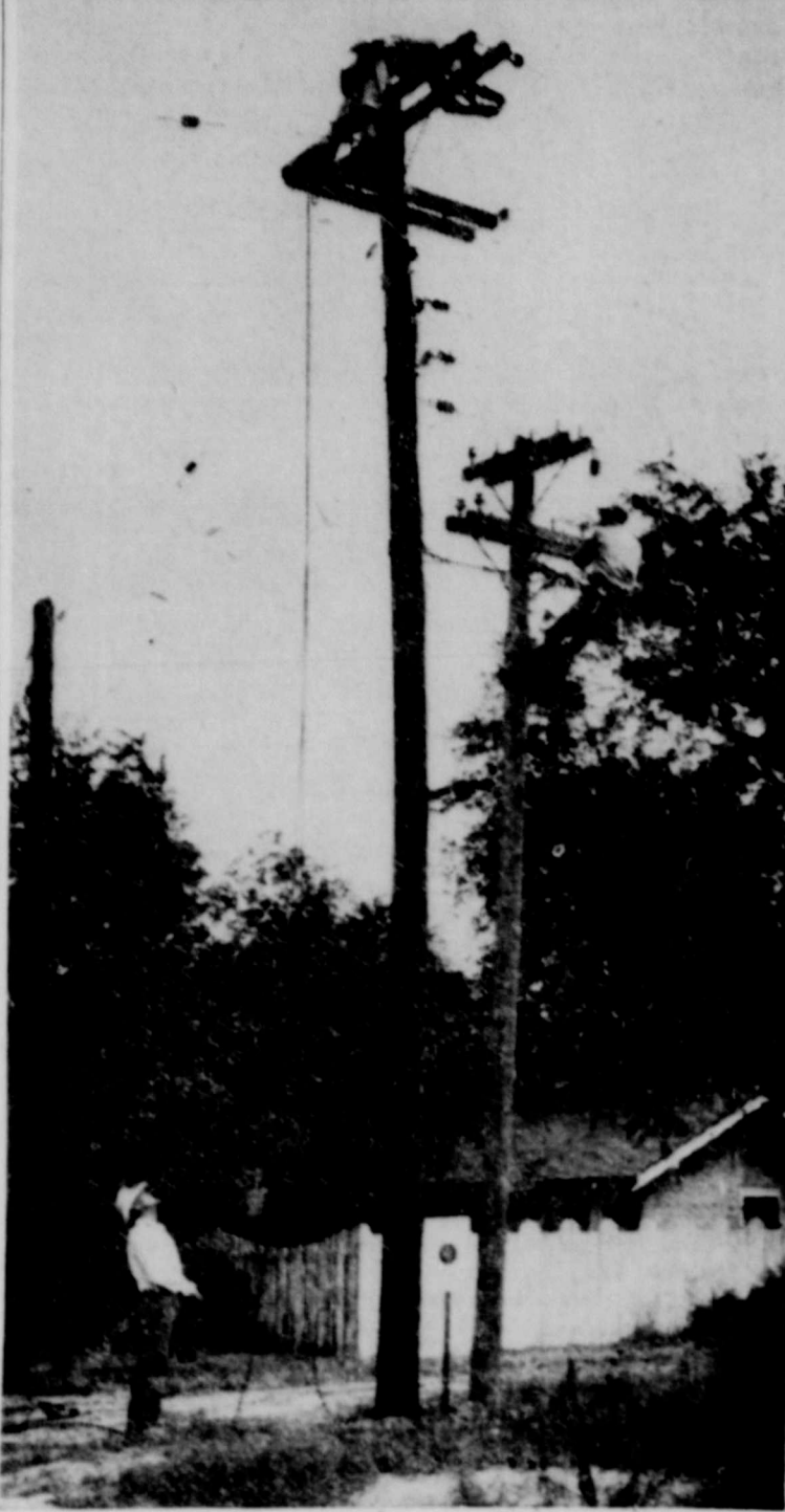
IMPROVE ELECTRICAL LINE — Members of a Community Public Service line crew are shown above installing new wire on 6th Avenue between Eton and Fordham streets. The old line from 6th avenue to 10th is being rebuilt and a new line to serve the new Stark addition is being installed from 10th to 16th ave. Shown l to r are K. S. Kutch (on the ground), and Troy Morris and George Symons atop the poles.
