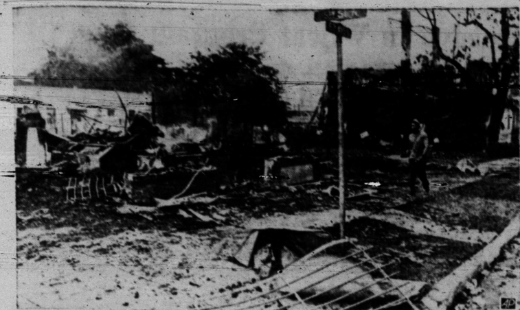
WHERE RIOTERS STRUCK —Smoldering ruins are all that remain at this street corner in Birmingham, Ala., following rioting in the Negro section. Looting and arson followed two bombings of Negro establishments. (AP Wirephoto)
