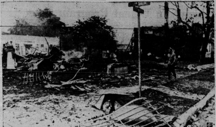
WHERE RIOTERS STRUCK—Smoldering ruins are all that remain at this street corner in Birmingham, Ala., following rioting in the Negro section. Looting and arson followed two bombings of Negro establishments. (AP Wirephoto)
