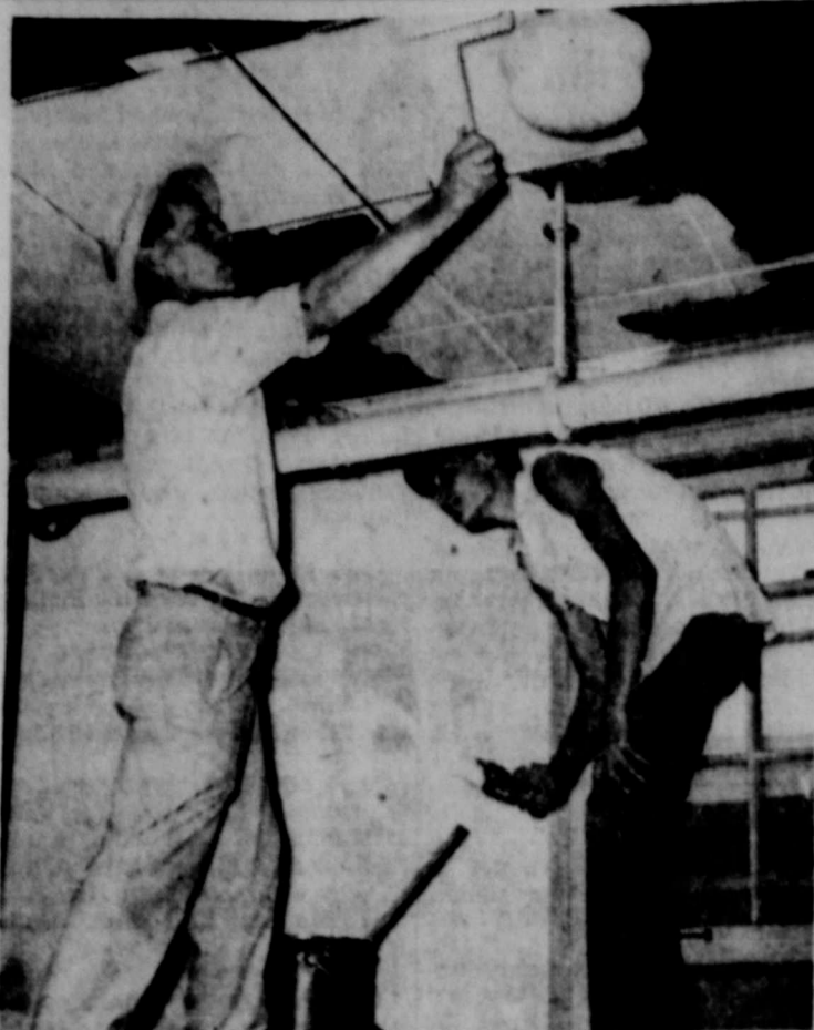
SUMMER REPAIR JOB—Oliver King, left, and Charles Smith have been hard at work this summer at the school building getting ready for the new school term and one project is the remodeling of the band room. New insulation board is being put on the walls and ceiling and the room is getting a new coat of paint.
