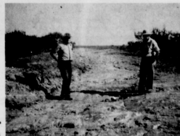
HORACE PADGETT, (left) and Nolen Bird, Soil Conservation Service technician, observes a newly constructed diversion terrace on Padgett's farm. The diversion diverts about 700 acres of drainage away from one of his cultivated fields. This outside drainage has caused severe soil erosion on the cultivated field. Padgett reported the diversion worked to perfection during the recent heavy rains and no damage was done to his valuable cropland.
