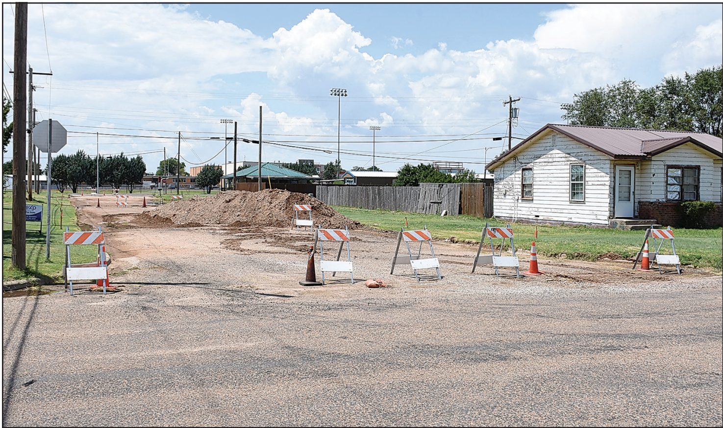
New Paving Project — Construction on 7th Street between Grand Avenue and Ashland Avenue is underway. In the coming weeks, Bermea Construction will soon be adding curbing and pavement to the street.
