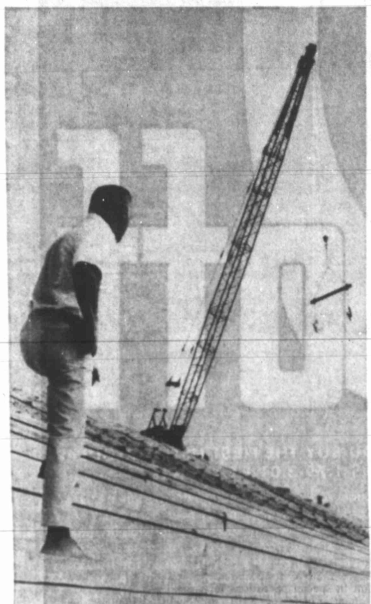
IT'S COMING ALONG — Leo Margolian, general manager of Texas International Speedway near Bryan, observes the progress being made on the concrete grandstands.
