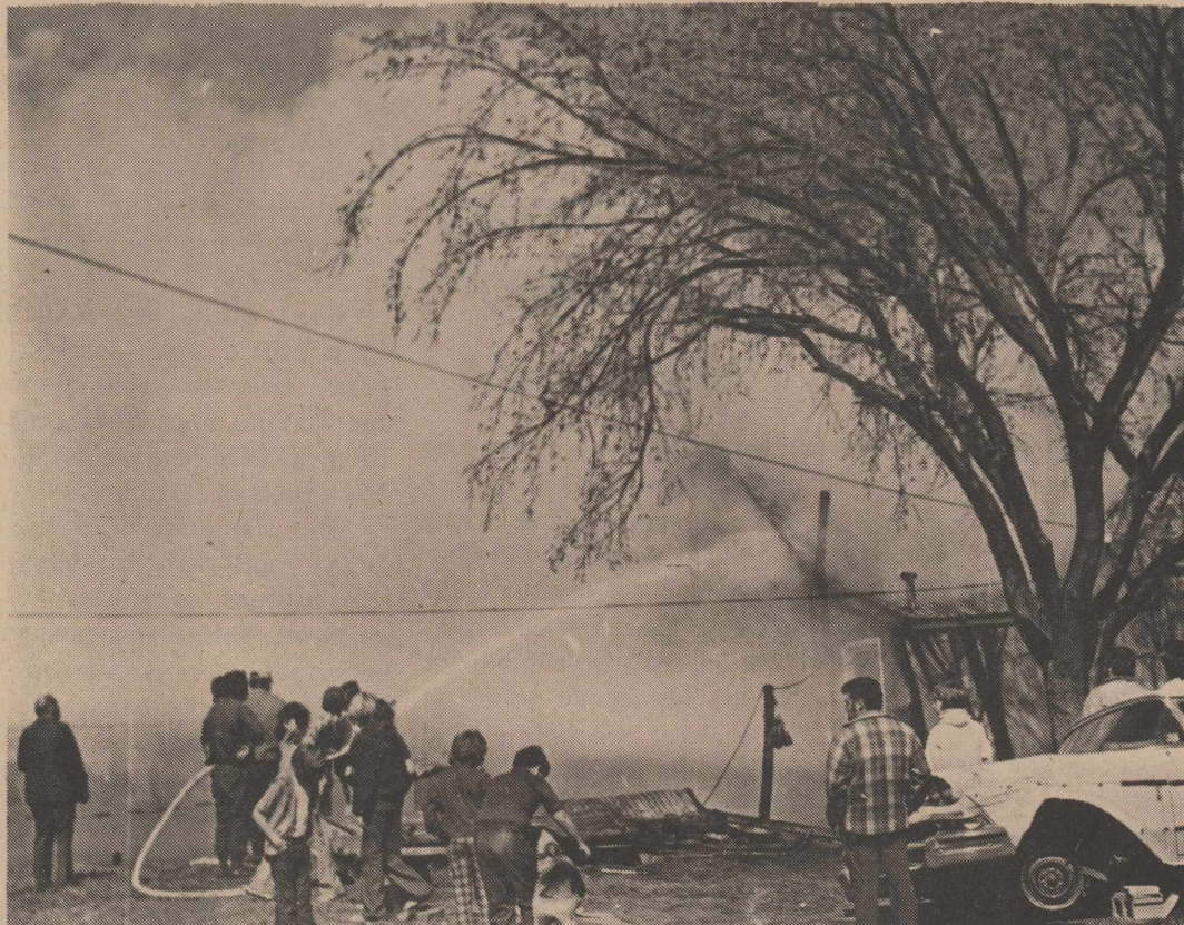
FIRE DESTROYS HOME
