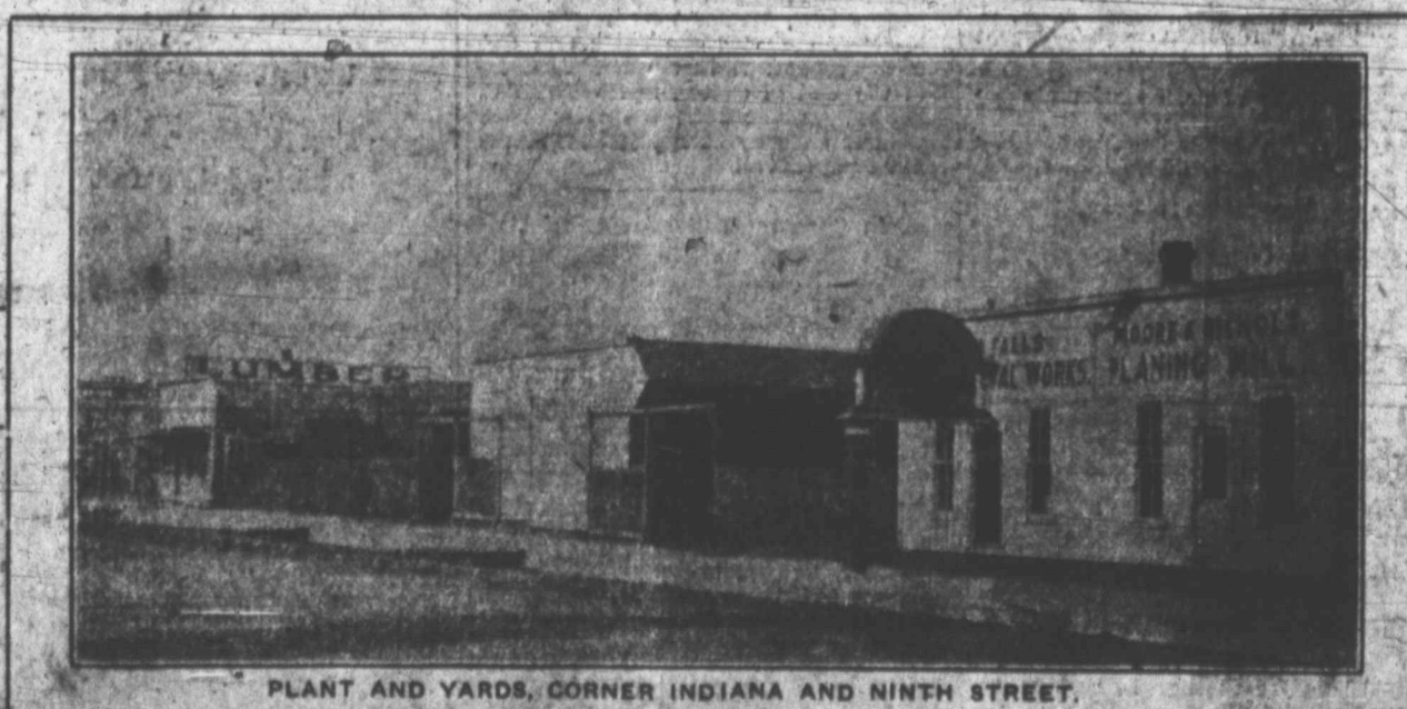
PLANT AND YARDS, CORNER INDIANA AND NINTH STREET.
