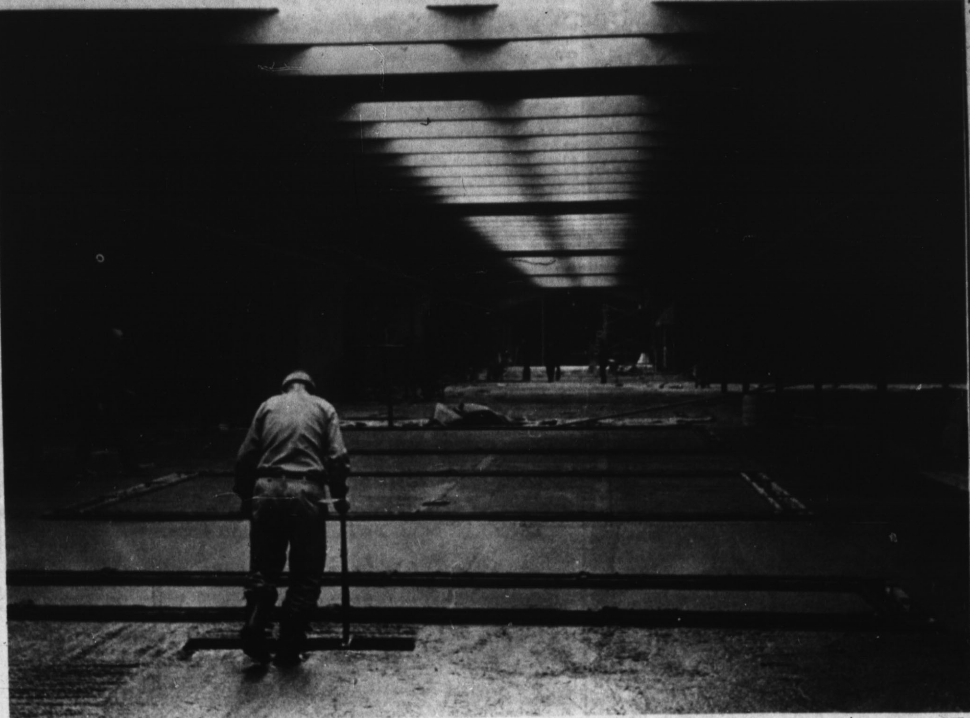
INSIDE WORK PROGRESS —Work on the Sugarland Mall north of Hereford round. The building will house numerous businesses including the already complete Furr's. (Staff Photo by Wain Miller)
