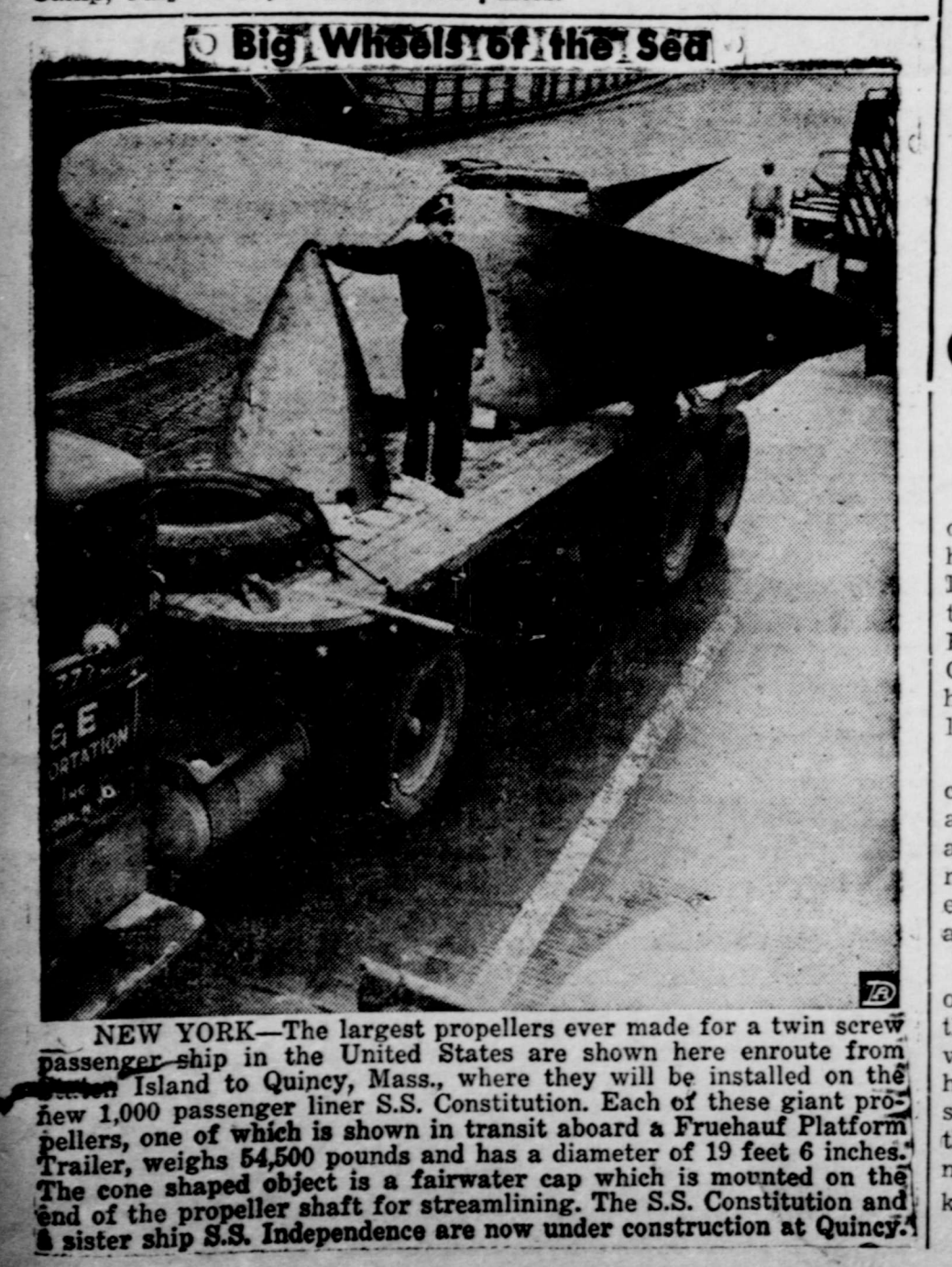
NEW YORK—The largest propellers ever made for a twin screw passenger ship in the United States are shown here enroute from Quincy, Mass., where they will be installed on the new 1,000 passenger liner S.S. Constitution. Each of these giant propellers, one of which is shown in transit aboard a Fruehauf Platform Trailer, weighs 54,500 pounds and has a diameter of 19 feet 6 inches. The cone shaped object is a fairwater cap which is mounted on the end of the propeller shaft for streamlining. The S.S. Constitution and a sister ship S.S. Independence are now under construction at Quincy.
