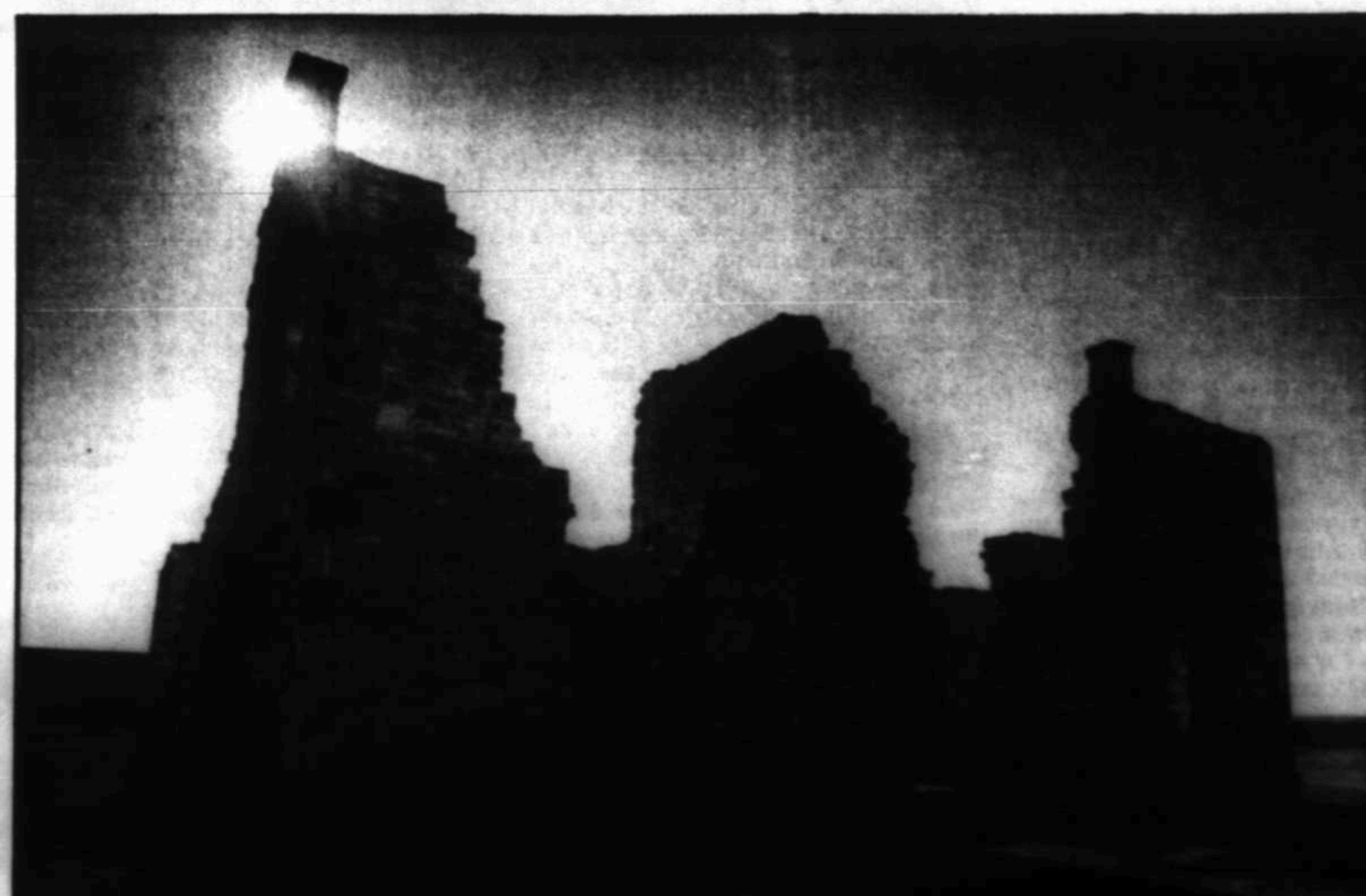
Park rangers and rock masons labor to reconstruct married officers' quarters at the fort. Fifteen buildings at the historic site have been restored (top). The shell of the commanding officer's home is the only two-story building at the site.
