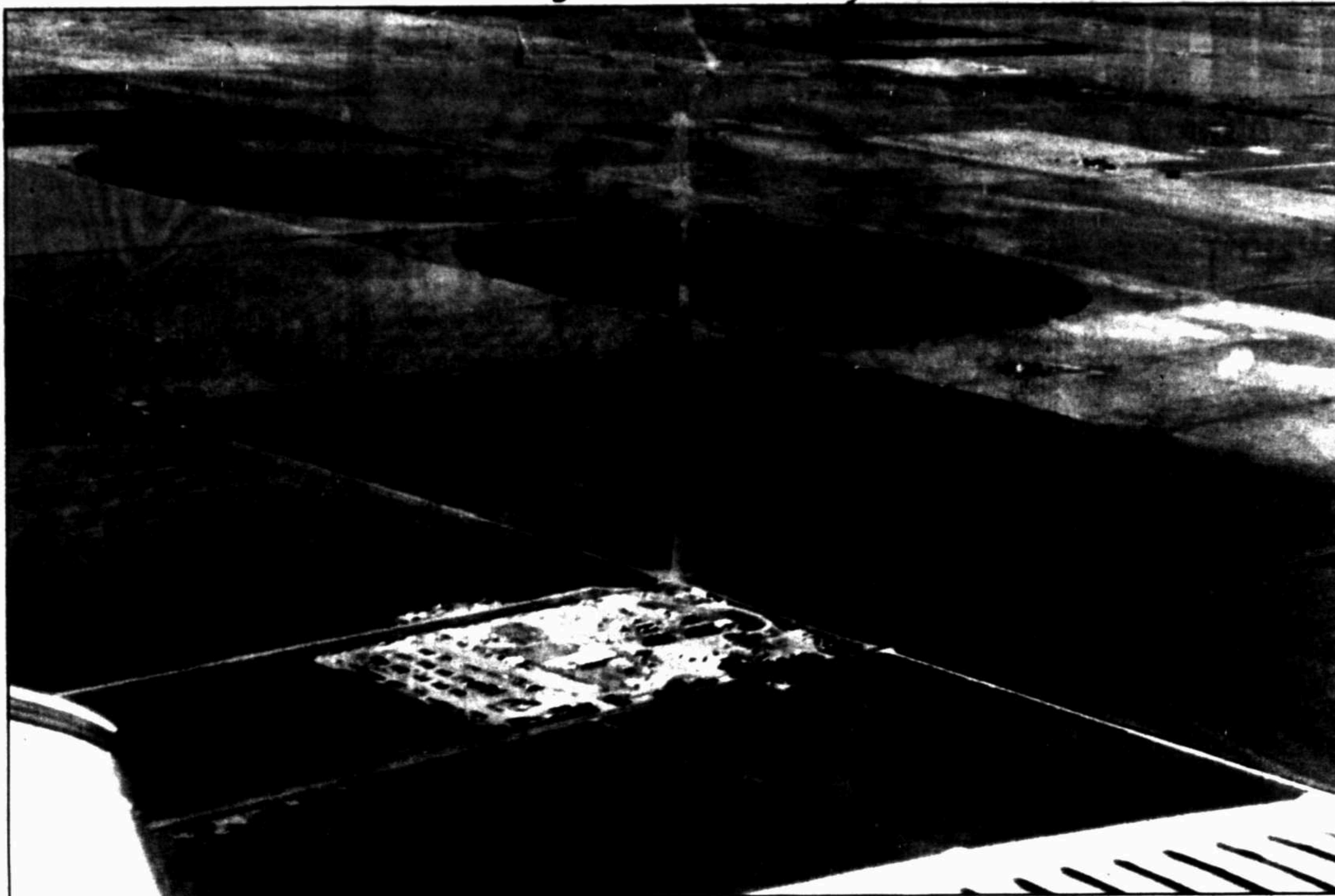
The terminal point of the Transpetco Pipeline, left top, currently serves the Postle-Hogue field in Oklahoma but is ready to expand into Kansas. The move would open the Mid-continent area to CO2 recovery. The pipeline under construction, below left, has the capacity for 200 mmcf but has been delivering only 60 mmcf to Mobil. While Mobil plans to take another 30 mmcf within the next few months, the line will still have plenty of capacity to serve other projects. Transpetco has identified over 100 fields in Texas, Oklahoma and Kansas as potential CO2 candidates for the pipeline.
