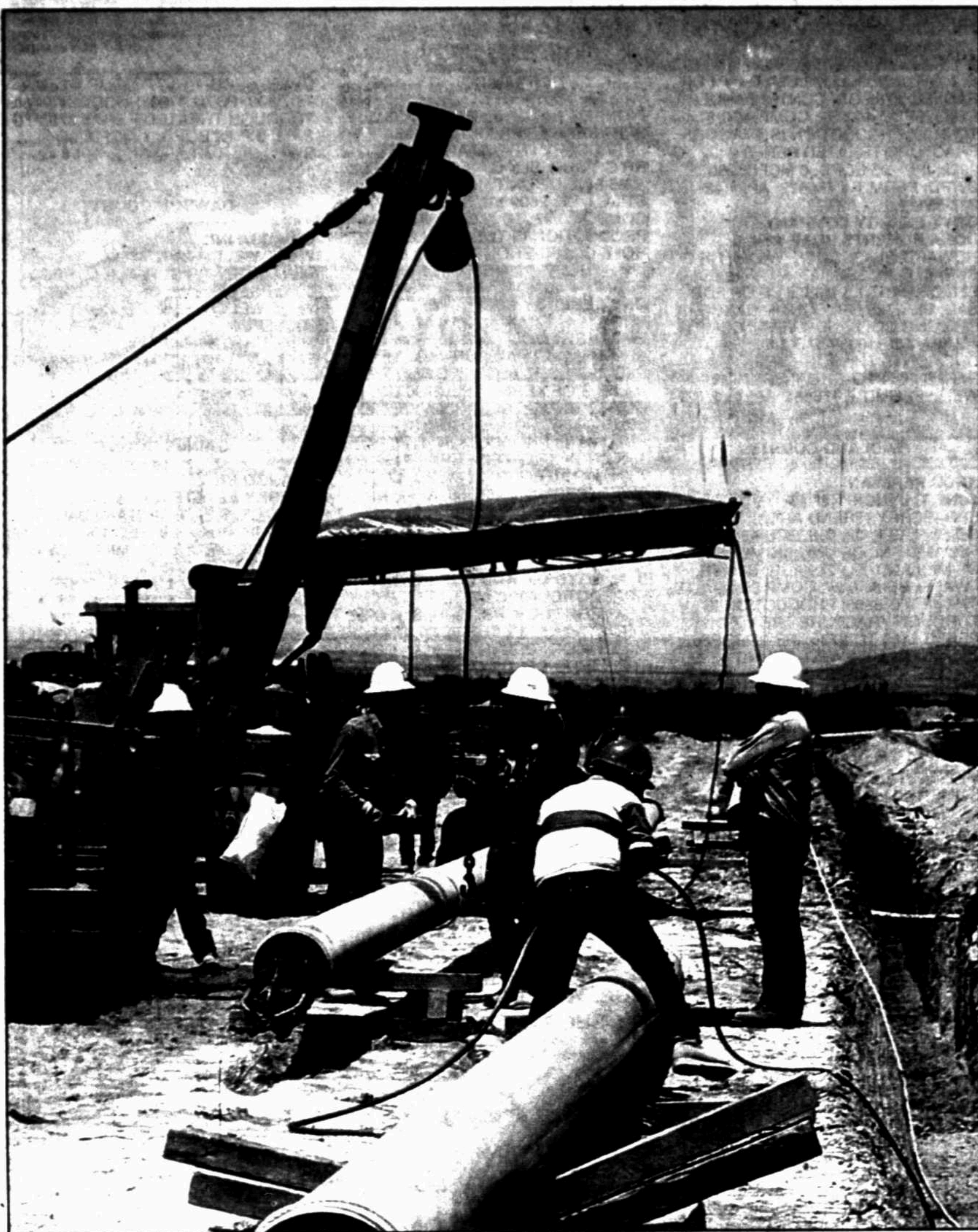
Workmen, above, complete a 15-mile pipeline expansion in the Val Verde Basin, where pipeline activity has proliferated. PetroSource announced a new CO2 pipeline that will provide Val Verde CO2 to projects in the Basin.
