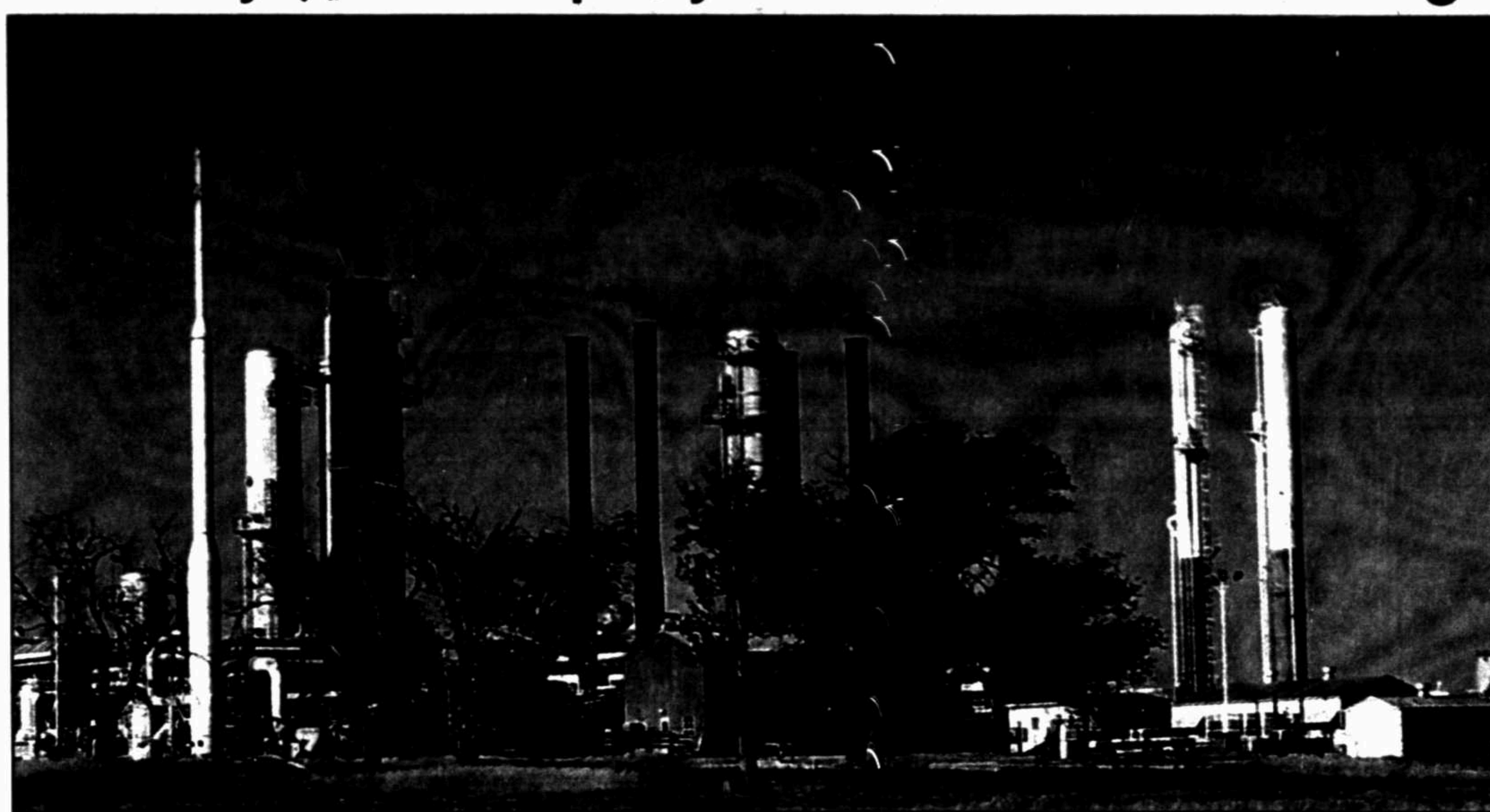
A gas processing facility in the SACROC area, photographed in the 1980s. The first major CO2 project in the Permian Basin had a colorful beginning that made it a first in several categories. Pennzoil, which purchased Chevron interests in the unit, is now exploring plans to upgrade the CO2 recovery aspect of the giant Canyon Reef producing unit.
