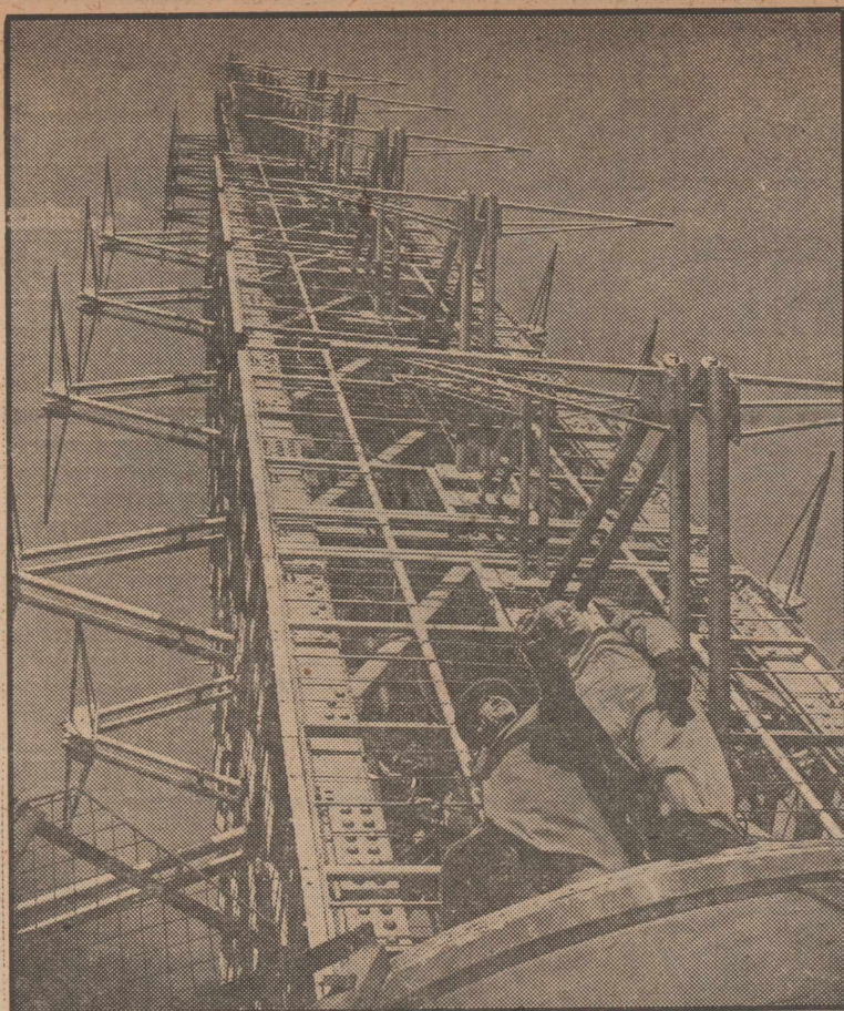
VIDEOZONE —High above New York City, two radio experts hold a conversation at the base of the Empire State Building television antenna mast. Final grid—last large structural piece to be added to the tower, completing it except for wiring—when installed, should make the video antenna ready for broadcasting early in December, 1951.
