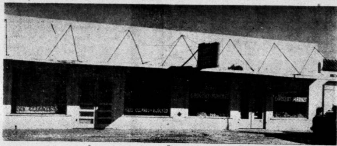
Above are pictured the firms owned by Leonard Scott, which includes Scott's Cleaners & Laundry and Scott's Cash Grocery, which are located 1-2 block south of the City Hall. The cleaning shop offers a variety of services. They have a cold storage vault, will block and clean hats, do laundering and dry cleaning, as well as handle made to measure suits. In the grocery you will find a complete line of quality foods and meats.
