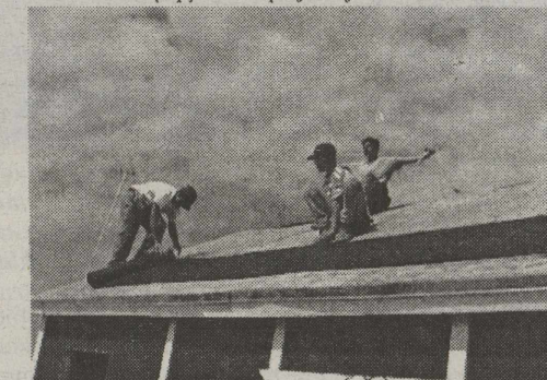
Colt Smith, Zach Burson and Max Comer work on the roof together.
