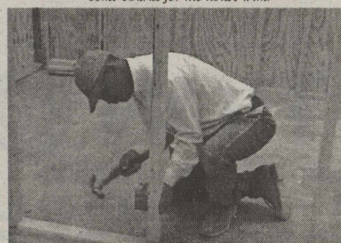
Bryan Burson prepares the house for electrical wire.
