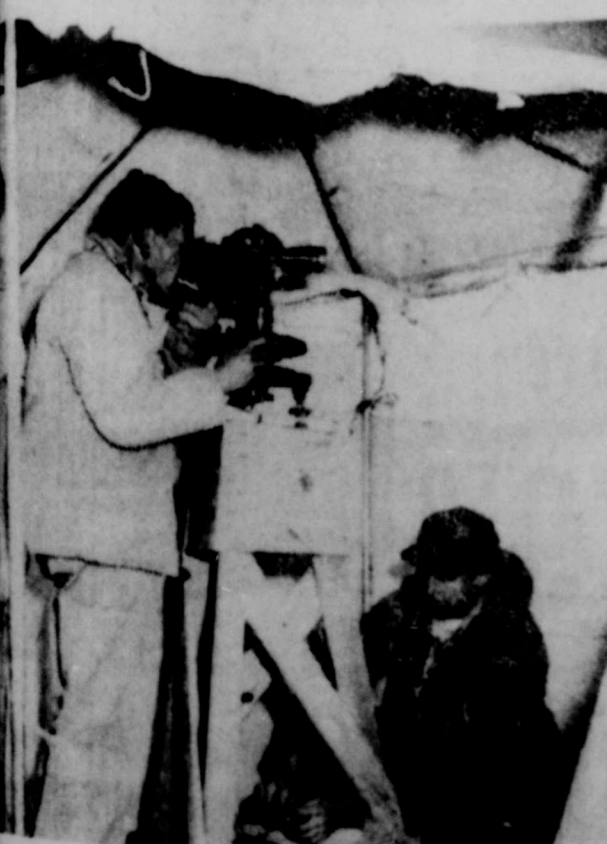
PARTY AT WORK—W. M. Johnson, left, and Dick Haney carry out their part of a geodetic survey. The through which Johnson is looking is a theodolite, and he's on top of towers 8 to 15 miles away. The angles of the towers are recorded, and by computation, the distances are measured. Particular tower was located 2 miles northwest of Lipscomb.
