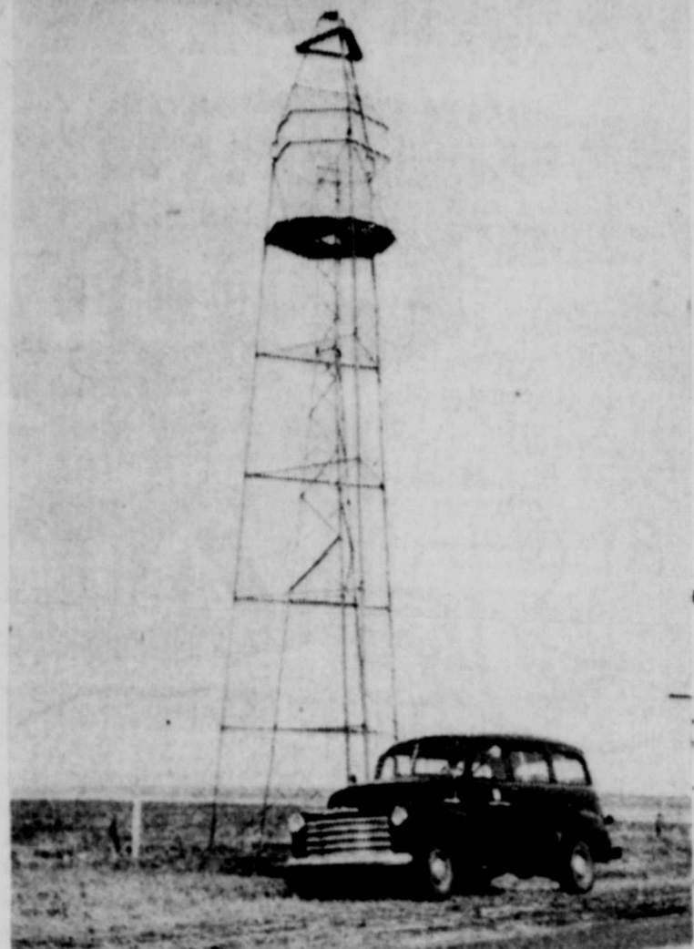
STEEL TYPE TOWER—This 37-ft. steel tower is used by the geodetic survey party when they need to get higher off the ground than they can go with a wooden one. These steel towers come in 37, 64, 77, 90, 103 and 116 foot heights, and a steel tower crew can erect one in less than a day. This one is located two miles east of Darrouzett. Both the light and the observation party use the tower.
