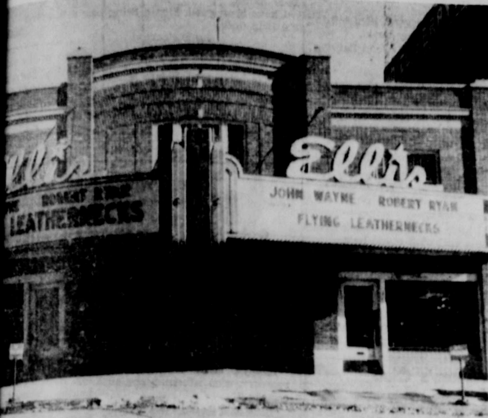
SED UP—The Ellis Theatre blossomed out with a real "new look" this week with the addition of a marquee across the front. This porcelain and glass marquee is 50 feet across and 12 feet high. It is made of neon tubing, scores of flashing lights, and 16 floodlights on it. The large red letters on the lighted white background with each change of picture at the theatre.
