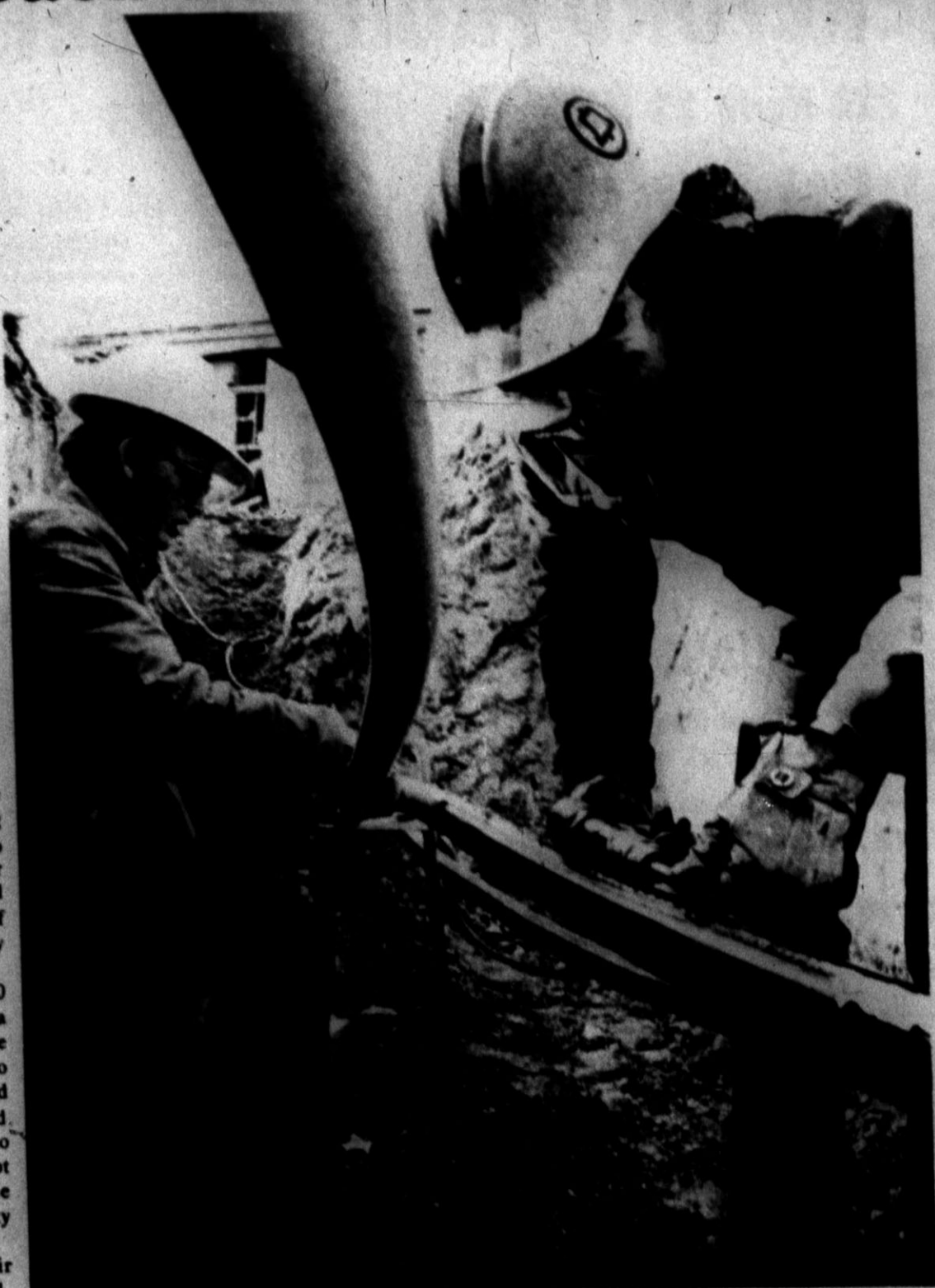
Two cable splicers work on buried cable to provide hundreds of additional circuits—protected from ice, hurricane or tornado.
