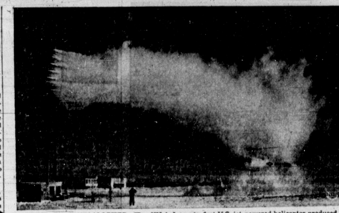
ICING ON A HELICOPTER — The HU-1 Iroquois, first U.S. jet-powered helicopter produced for the military, hovers in an artificial ice cloud in Ottawa. The icing spray rig, operated by Canada's National Research Council, has 143 spray nozzles mounted atop a 50-foot steel mast. The amount and size of the ice droplets can be controlled. The Iroquois, manufactured by Bell, has also undergone cold-weather tests in Alaska and desert tests in Arizona.
