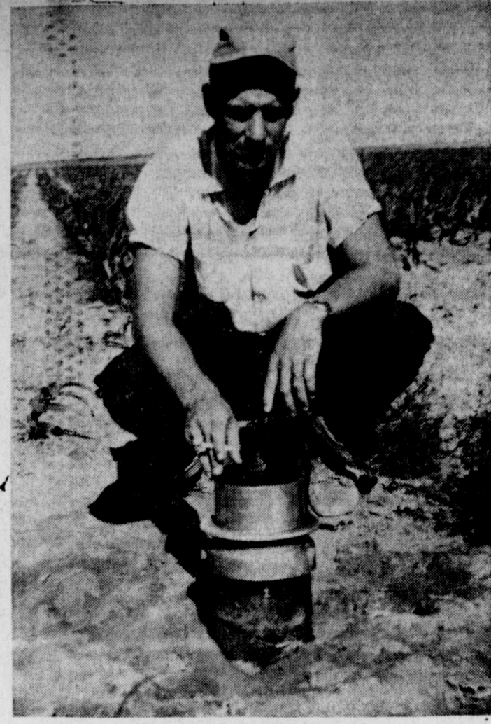
ON STEEL PIPE underground sprinkler line, is shown by Gene Hamilton, operator of the T. L. Timmons farm where the sprinkler system was installed. See story on Page 1, Section 3.
