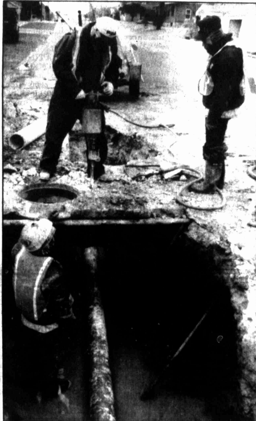
City of Big Spring workers use a jackhammer to remove concrete above an eight-inch sewer line that was replaced at the intersection of Sixth and Main streets Tuesday. A tile storm drain above the line will also be repaired during the project.
