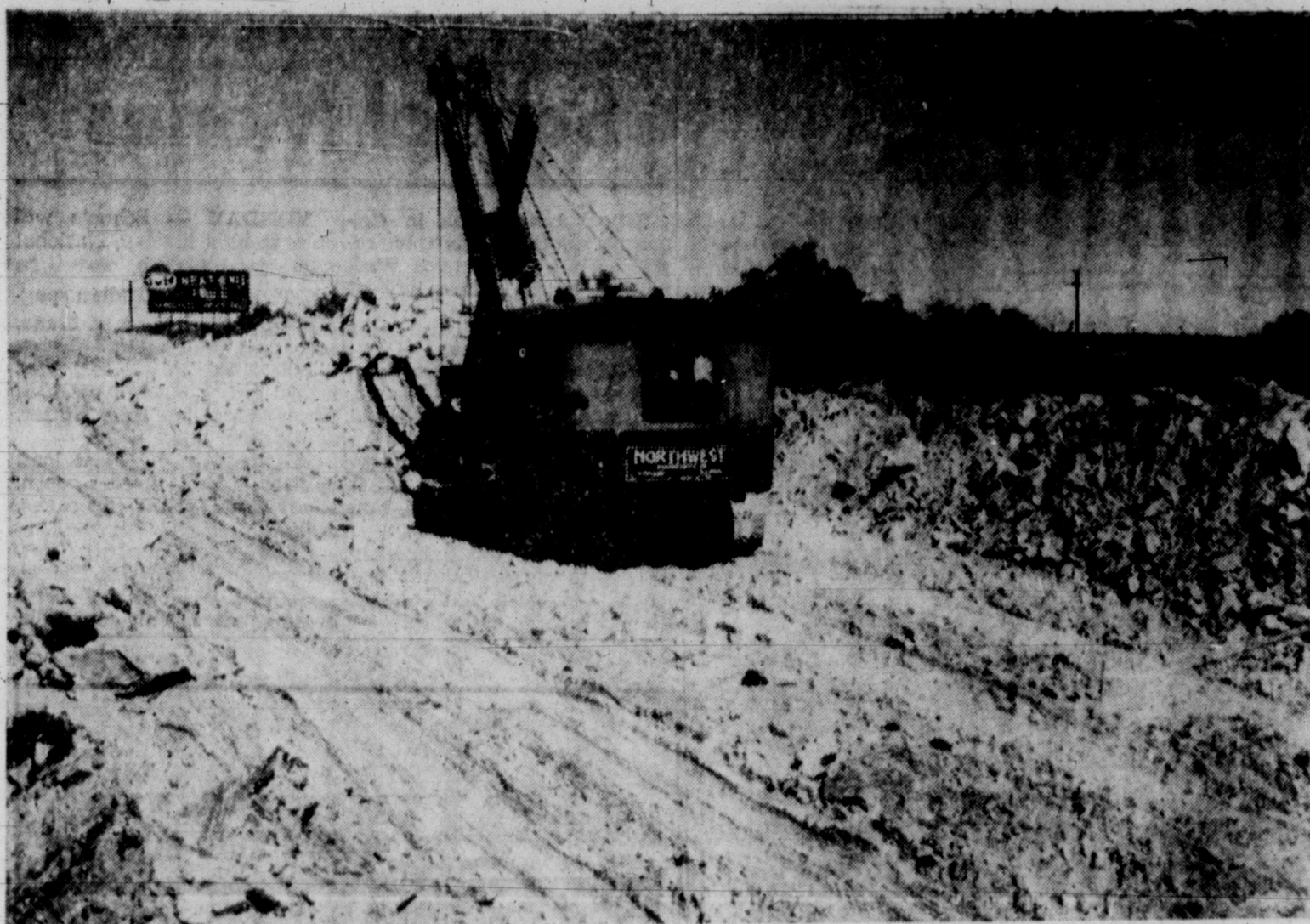
Service Road Construction
