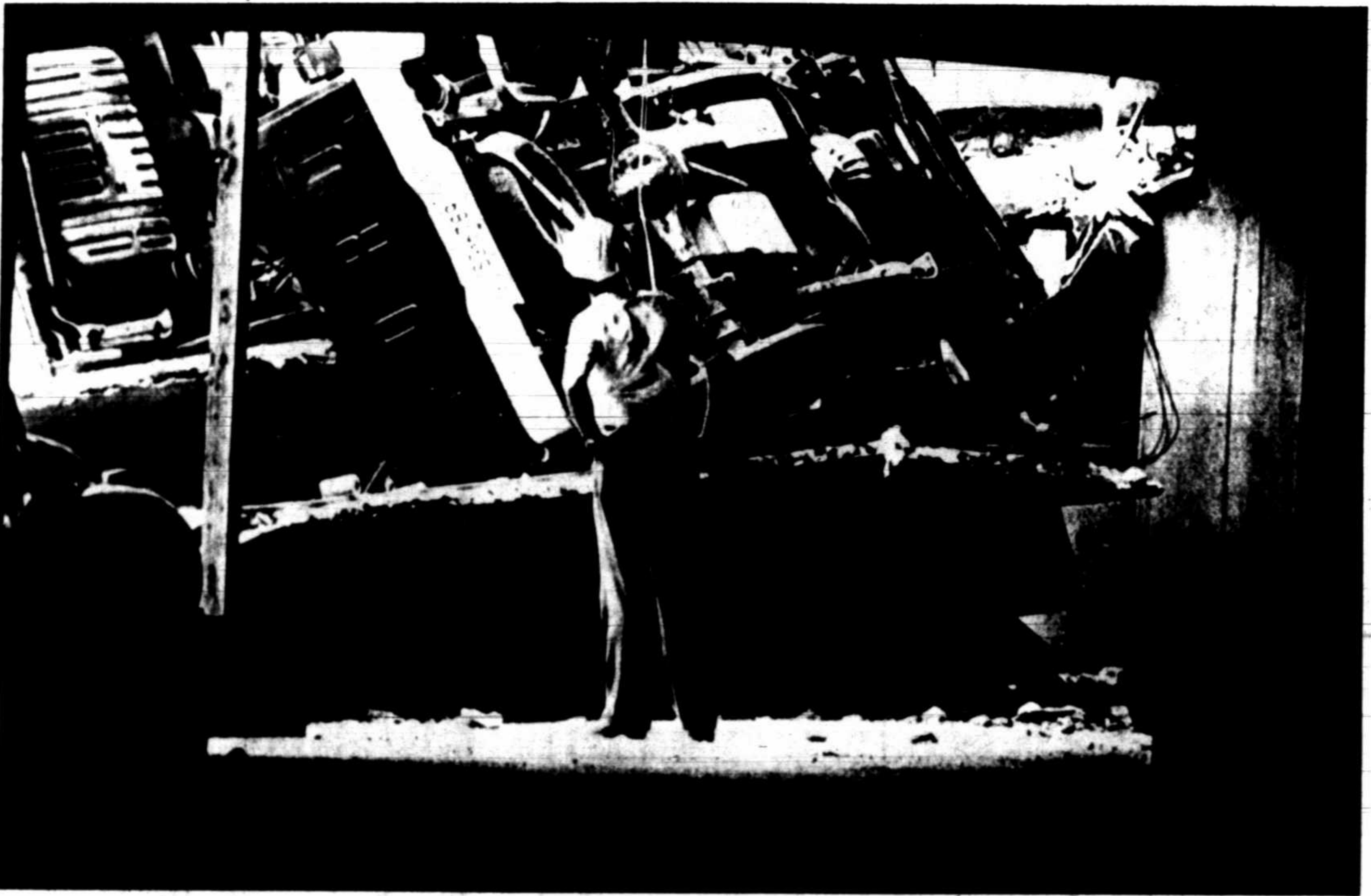
A rescue worker looks over crushed cars and trucks Tuesday in north Houston after a section of the Continental Bank Parking Garage collapsed. No one was injured in the cave-in.
