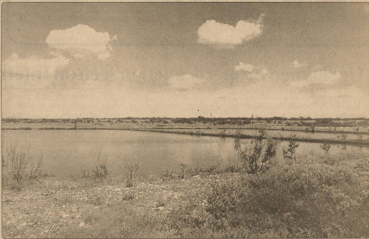
photo by Kathy Mankin Wastewater treatment plant — The City of Eldorado's sewer plant consists of three ponds covering more than 19 acres along the eastern edge of town. Last week the city was cited by the Texas Natural Resource Conservation Commission for non-compliance with state discharge standards. City officials say the problem is an ongoing one and blame it on hot weather which stimulates the growth of algae in the ponds.
