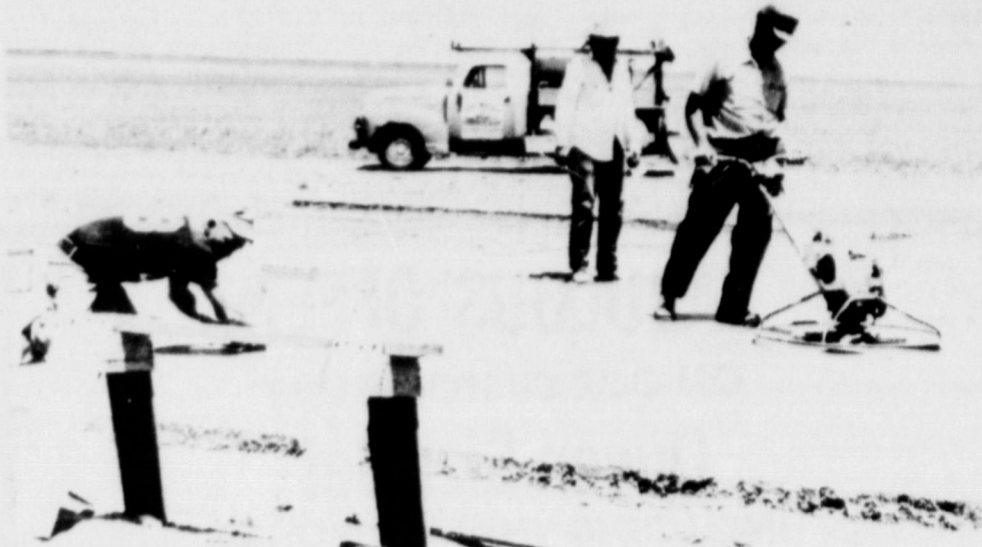
CONSTRUCTION UNDERWAY on the Terry Bridge Memorial Recreational Playground. Seen here is Toby Walker of Toby Walker Concrete and Monument Company in Littlefield and his employees, Bob Dillard and James Ball. As they smooth out the concrete slab for the tennis court.
