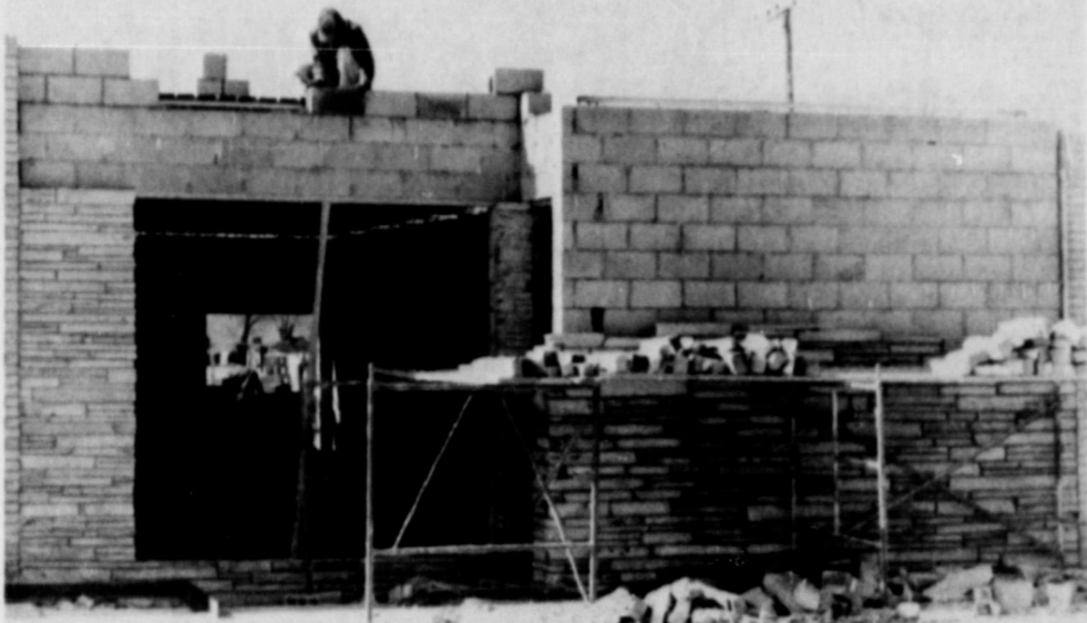
CONSTRUCTION BEGAN LAST WEEK on the new $16,000 Earth News Office plant, located adjacent to Rutlerford and Co. on main street. The 25 x 75 building is being constructed by Highlight Homes, Inc. and will be completed within the near future. The building will feature 2 offices, a lobby, workshop, 2 restrooms, darkroom and storage room. The front of the building is constructed from Arkansas Rock...
