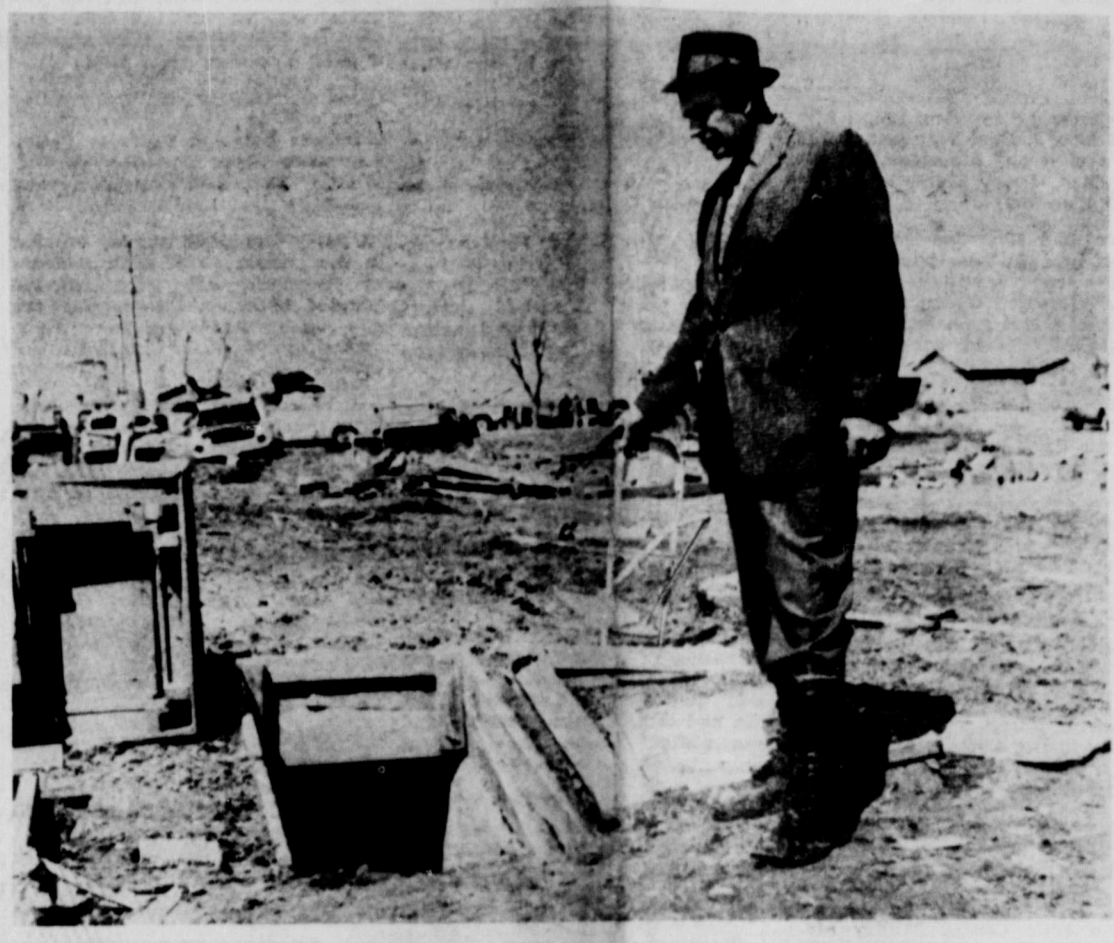
DOC MILLER OF OLTON POINTS TO THE STORM CELLAR — That saved many lives in Tuesday night's storm as people sought shelter from the storm. The cellar was packed to capacity during the height of the storm. Mr. Miller had this shelter to go to. (The door of the cellar was ripped frof its hinges.
