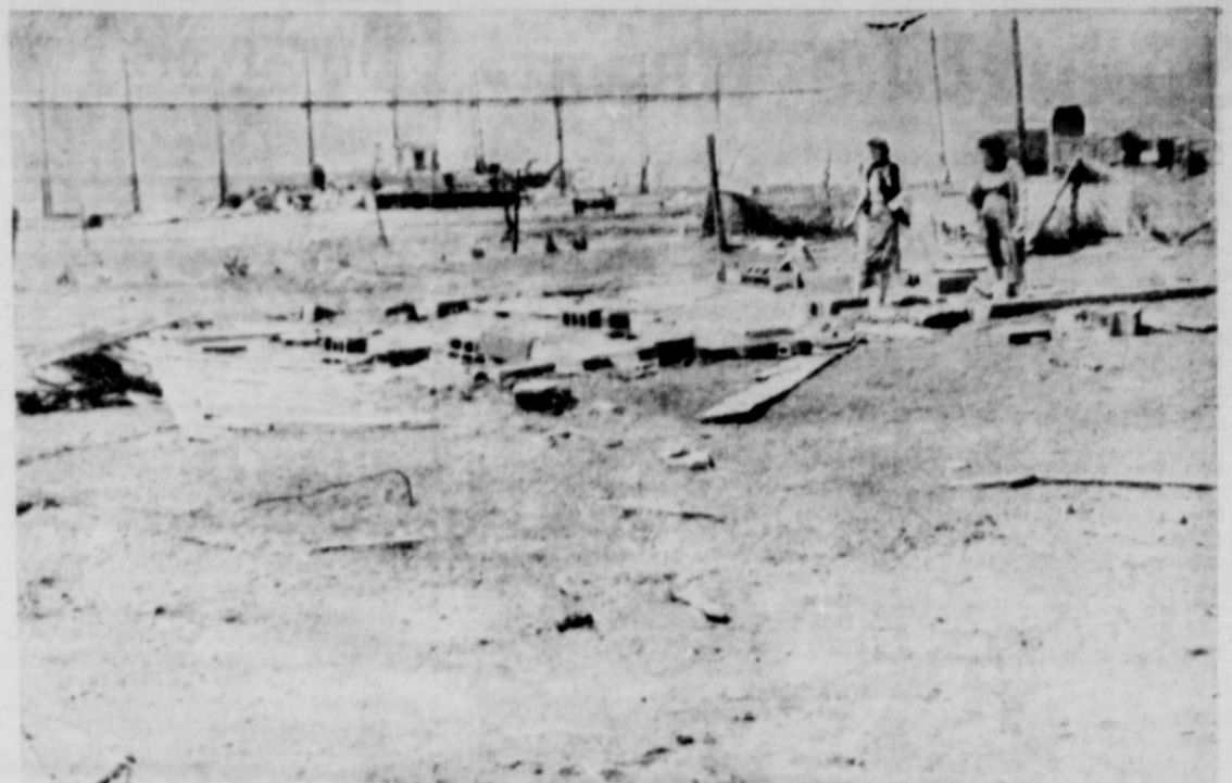
ONE KILLED AND ONE INJURED IN THE HOUSE THAT ONCE STOOD HERE — Only the foundation was left of the Earl Phelan home. The house was picked up and hurled approximately 500 ft. by the tornado. The body of Nona Beth Phelan was found in the debris. Mrs. Phelan was
