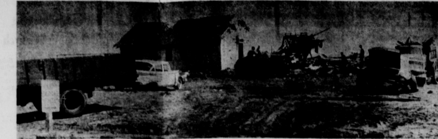
CLEANING UP OF THE SCATTERED DEBRIS - Was started early Wednesday morning when men along with a large number of others gathered with bulldozers and tractors to help friends of the small community to dig out from under the destruction. In
