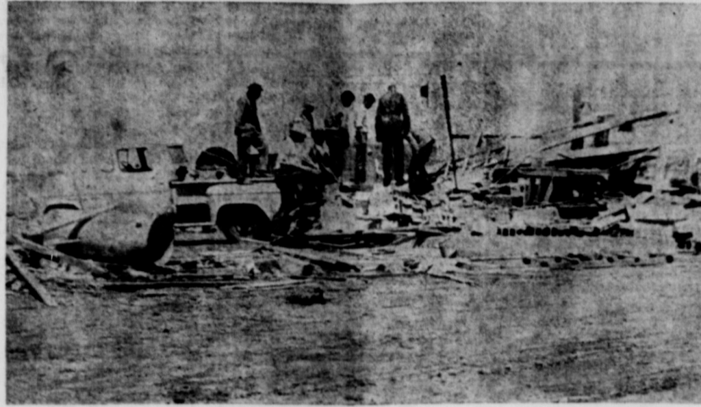
ALL THAT IS LEFT OF THE GIN OFFICE - Is one wall standing and debris piled everywhere. Residents of Sunnyside are pictured as they begin the cleanup of the debris Wednesday morning.
