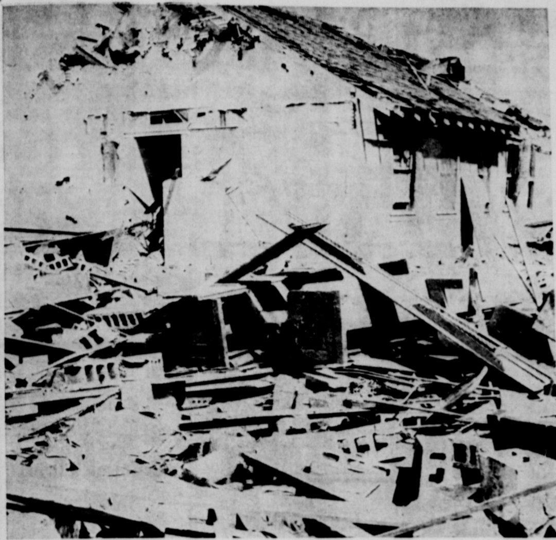
THE BAPTIST CHURCH IN SUNNYSIDE — In the foreground is the church auditorium which is left in debris. A Bible near what was the pulpit was left open at John 1:12. Pews were beat into the blocks. In this debris the body of J. B. Kidd,
