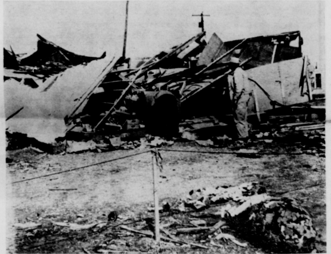
THE REMAINS OF SUNNYSIDE'S ONLY GROCERY STORE — Owned and operated by Mr. and Mrs. E. R. Sadler. The Sadlers had not closed the store for the evening, but when the atmosphere took on a noted change and a stillness hovered, they, their son, and Charles Hedrick, living in the adjoining quarters, fled to the car in an effort to get to their home and shelter one fourth mile away. However, the tornado was upon them and flipped their car over and over, landing it across the highway in the church parking lot among the masses of parked cars. Mrs. Sadler fell from the car and was among the injured. She is in the Castro County Hospital.
