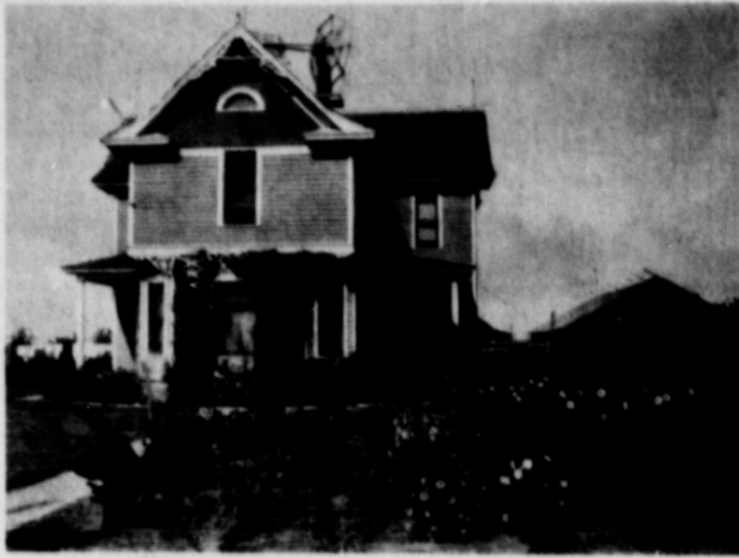
THIS HOME WAS BUILT in 1910 by Ray Axtell's father. It was located 2 miles west of Sunnyside. The Ray Axtells moved into it in the fall of 1939. It was torn down in 1947.
