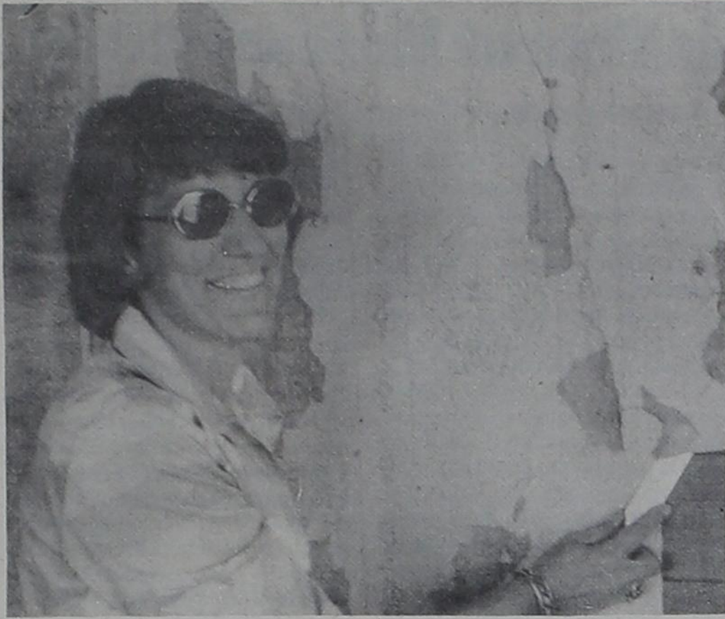
PEELING PAPER —Mrs. Betty Albers demonstrates the technique she uses to peel off layers of wallpaper in the Barton House at the Ranching Heritage Center. By removing the wallpaper piece by piece, Mrs. Albers discovered the original wallpaper that was in the house when built in 1909. (Times Photo)
