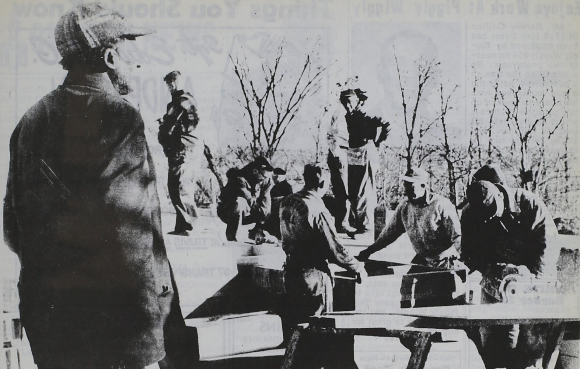
CHIPPING IN: When neighbors in Greenville, New York learned that 70-year old Moses Van Zandt's house was condemned to make way for a new road, they got together and built a new one.
