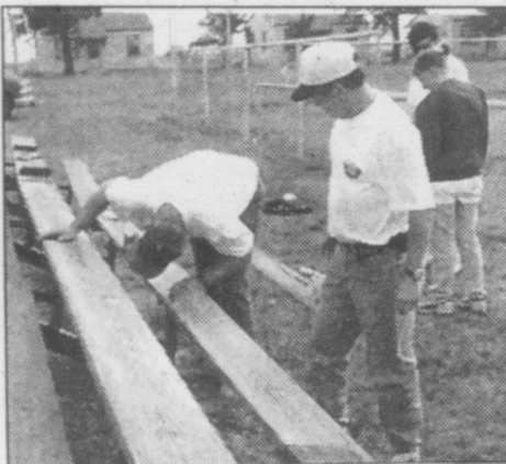
Forrest McLaughlin, inspects Jerry Ashford's work.
