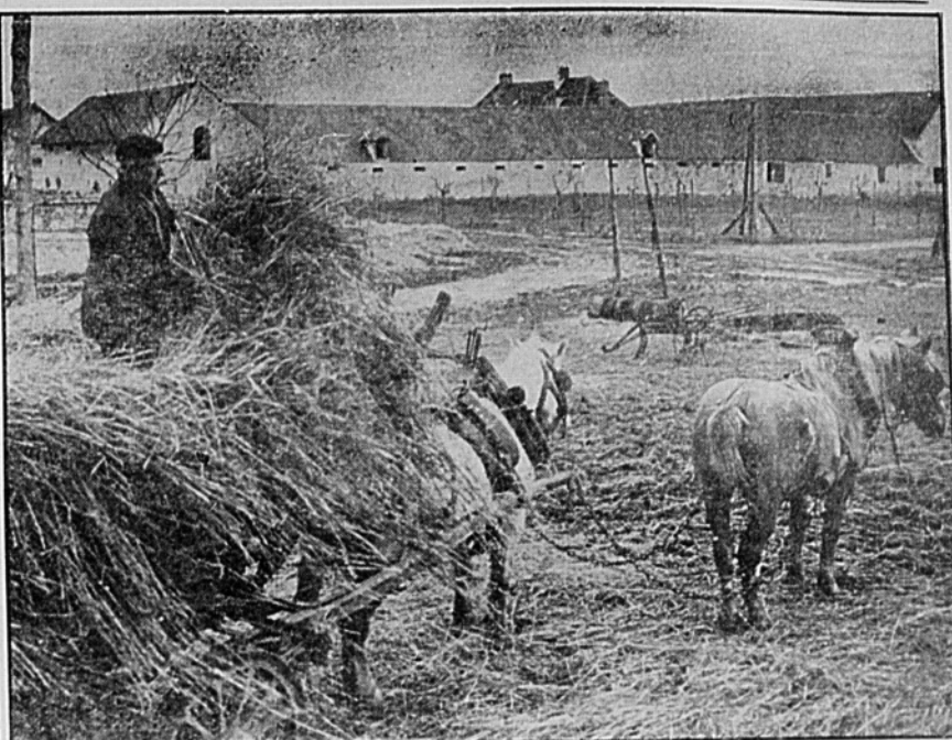
SITE FOR SHAPE —This quiet pastoral scene will soon become a beehive of activity as workmen move in to construct buildings for Supreme Headquarters, Allied Powers in Europe (SHAPE). Site is about 17 miles west of Paris and was personally selected by General Eisenhower, SHAPE's supreme commander. The tract takes in some 60 acres.
