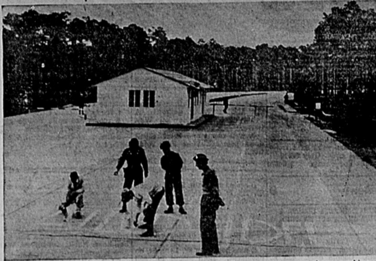
BERLIN—Under direction of Allied Military Personnel, German painters are shown marking out traffic lanes leading to Berlin control point of the Berlin end of the autobahn. Lanes are designed for control of American, French and British traffic between Berlin, which is in the heart of the Soviet Zone, and the Western Sector of Germany under Allied Control. Beyond checkpoint, where gates are down, is no-man's land between the Western and Soviet check points.
