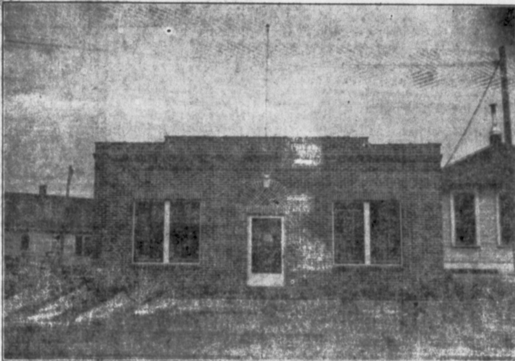
The $77,000 office building, shown above, is thoroughly modern in every way, and accommodates the latest and best equipment known in telephone science.
