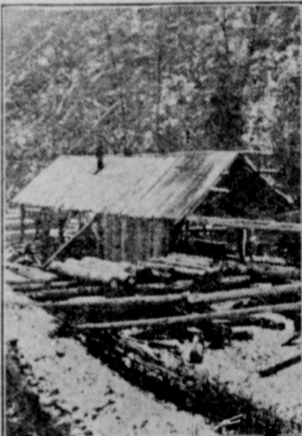
A Portable Sawmill in West Virginia Owned by Three Farmers Who Do Their Own Cutting, Hauling, Sawing and Selling, Working Only in the Afternoon—Its Capacity is About 3,000 Board Feet a Day, Cutting Mainly Hemlock, With Some White Ash.
