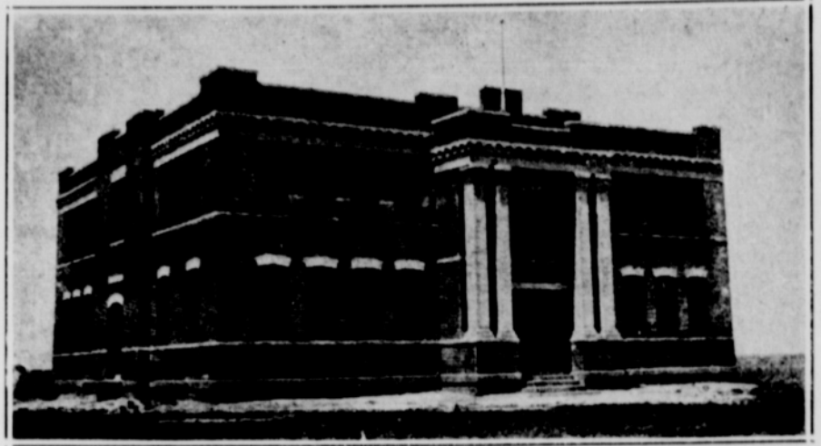
Slaton Public School Building, Built of Brick
