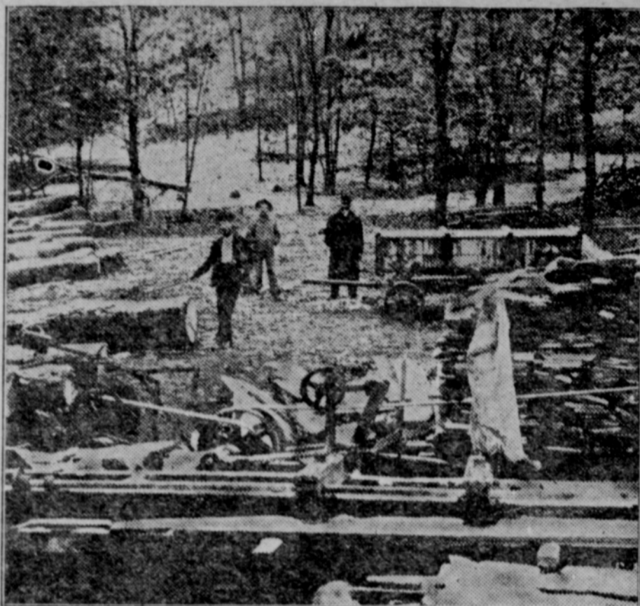
A Portable Sawmill Used for Converting Woodlot Timber Into Switch Ties, Which Are Extra Long—The By-Product of Such Ties in the Form of Slabs and Edgings, With Some Boards, Can Be Utilized for Lumber. Near Dubuque, Iowa.
