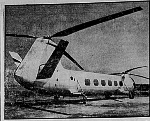
TWIN-MOTOR ROTOR CRAFT—Britain's first twin-engine helicopter, the "Bristol" type 173, is shown as it was unveiled for ground running trials in England. The super size ships, whose rotors are 48 feet in diameter, is designed to carry from 10 to 30 passengers or 2500 pounds of freight.
