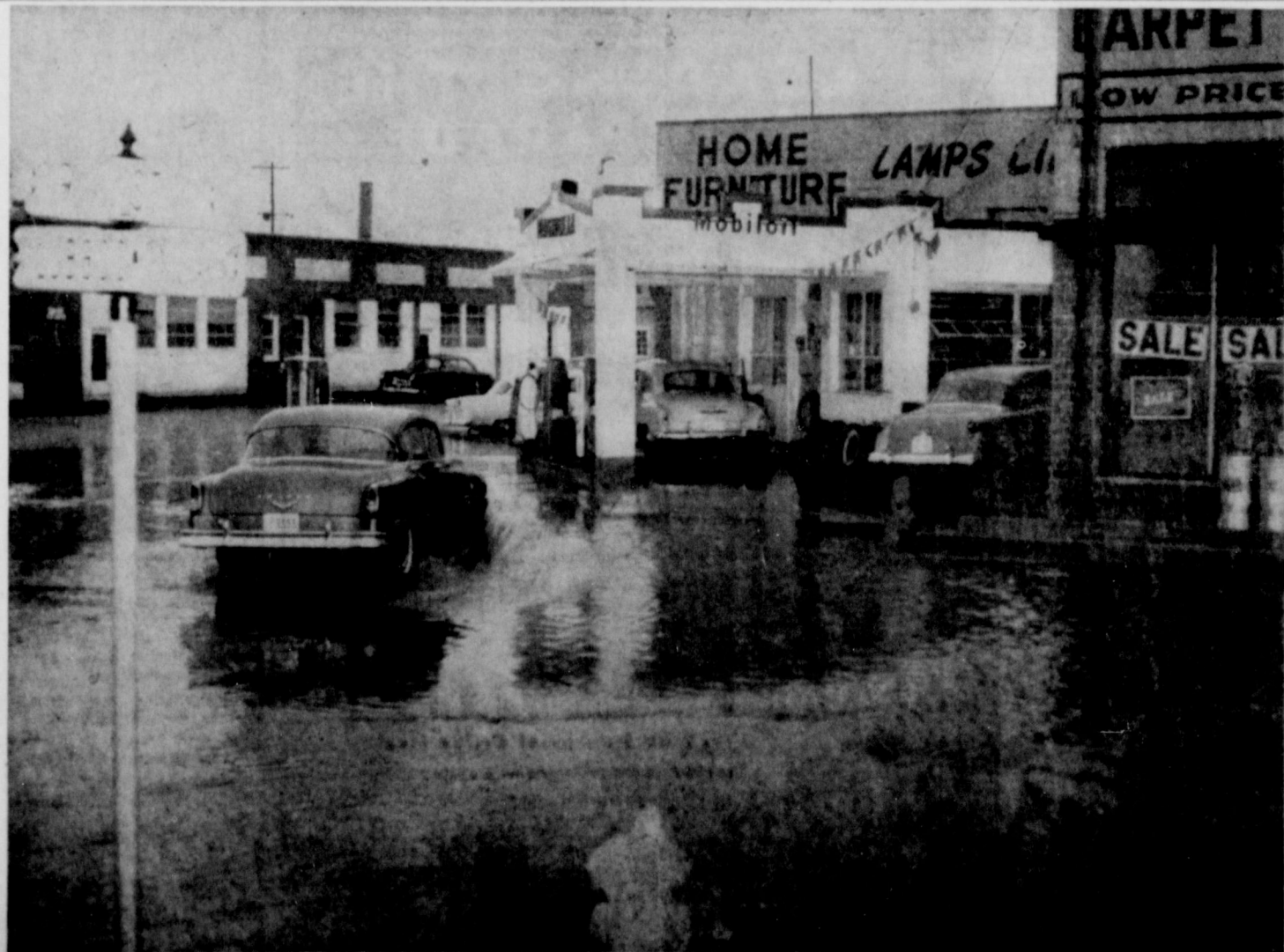
WET STREETS — The intersection of 9th and Lubbock streets was flooded Saturday morning by the heavy rains. Water completely covered the intersection, but did not stop traffic. Rains in Slaton amounted to about 1.3 inches, while
