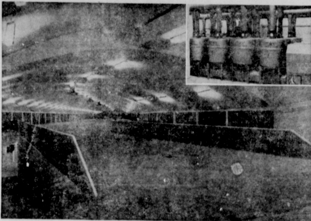
UNDERGROUND PARKING garage in Stockholm, Sweden, showing two levels in this vast dual-purpose civil defense shelter which can accommodate 10,000 persons. The garage, a key unit in the largest underground shelter program in the world today, is equipped with triple electric doors at the entrance ramp to wall out blast pressures, electric generators, and a special air filter system, (inset) to eliminate poison gas, germs and radioactive dust. (Swedish Civil Defense Photo)
