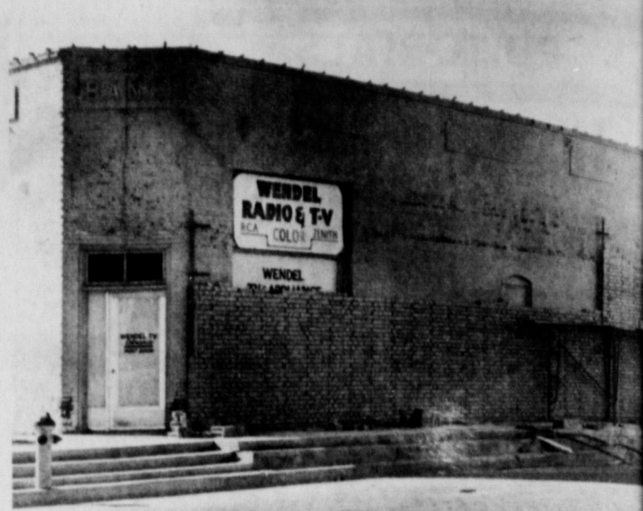
A NEW LOOK---The building on the corner of 9th and Garza Streets has new brick now. Wendel's T.V. & Appliances purchased the building and is still in the process of remodeling it. This picture was taken in the early stages of the bricking job. (SLATONITE PHOTO)
