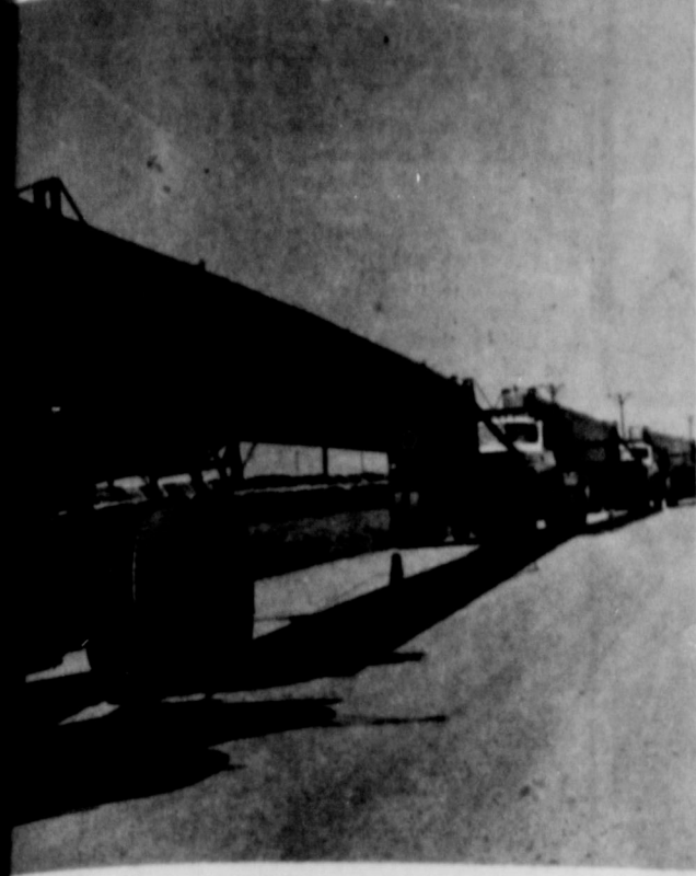
SS GOING UP---The new US-84 overpass over FM-41 on the west side of began to take shape this week with the erection of huge beams. Scenes here shows bringing in the big beams, one being hoisted into position, and workmen the beam into its resting place. The beams are 93 feet long and weigh 50,000 each. A total of 28 beams were required for the overpass--located between and Tom Sims Chevrolet at the west end of Division street.
