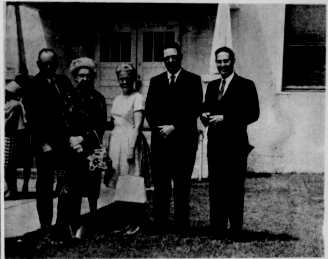
GROUND BREAKING--This picture, taken May 19, 1969, was the start of the new Educational Building for First Baptist Church of Slaton. Participating in the ceremony were Bill Alsbaugh, chairman of deacons; Mrs. Fred Stottlemire, a member of the church 53 years; Mr. and Mrs. William Jones, Sunday School and WMU leaders; and the Rev. J. L. Cartrite.
